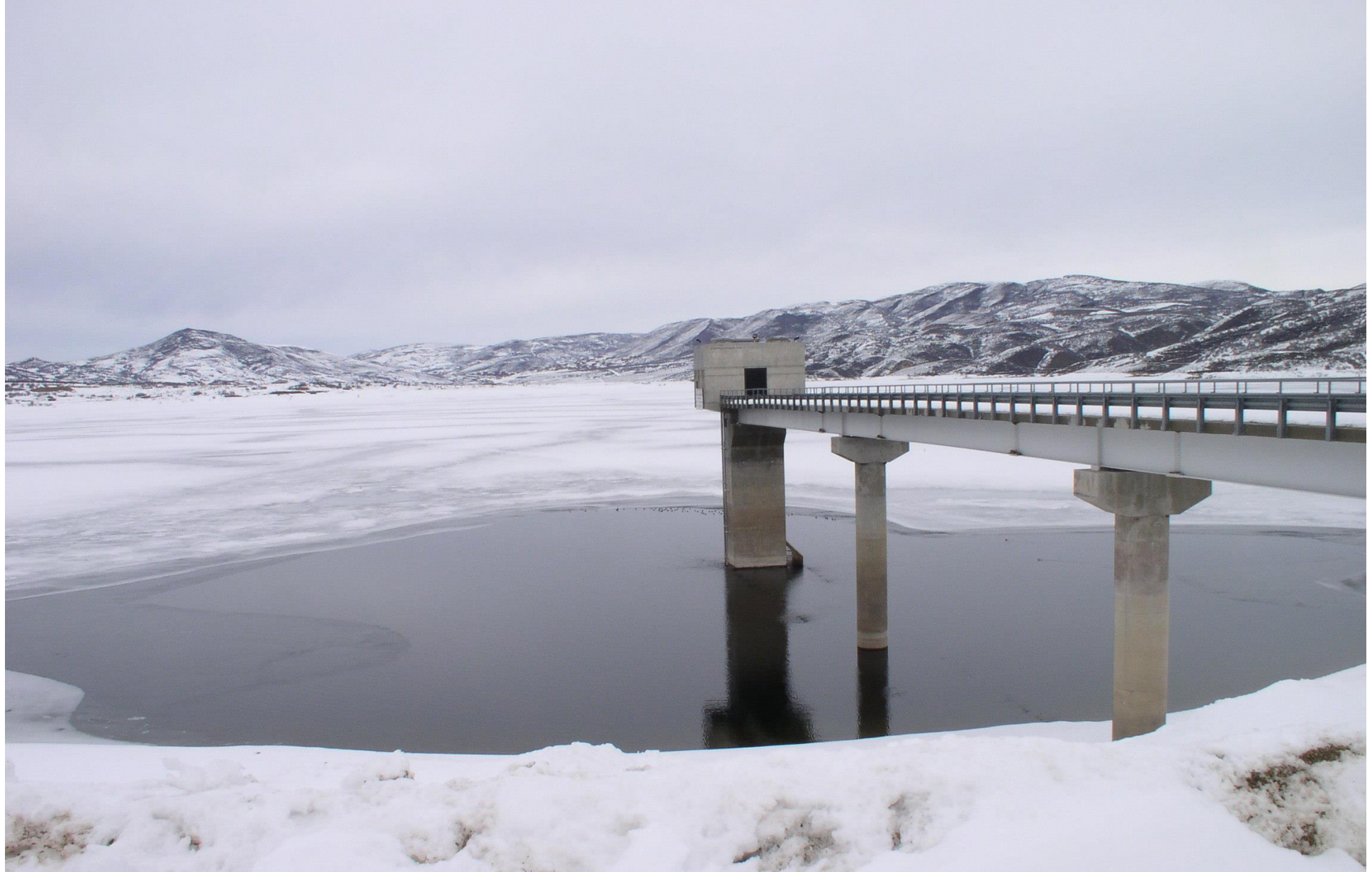
Jordanelle Reservoir Outlet Structure
