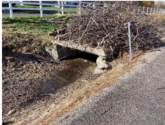
Photo 2-13: Vegetation Recently Removed from Bridge Culvert on South Jordan Canal
