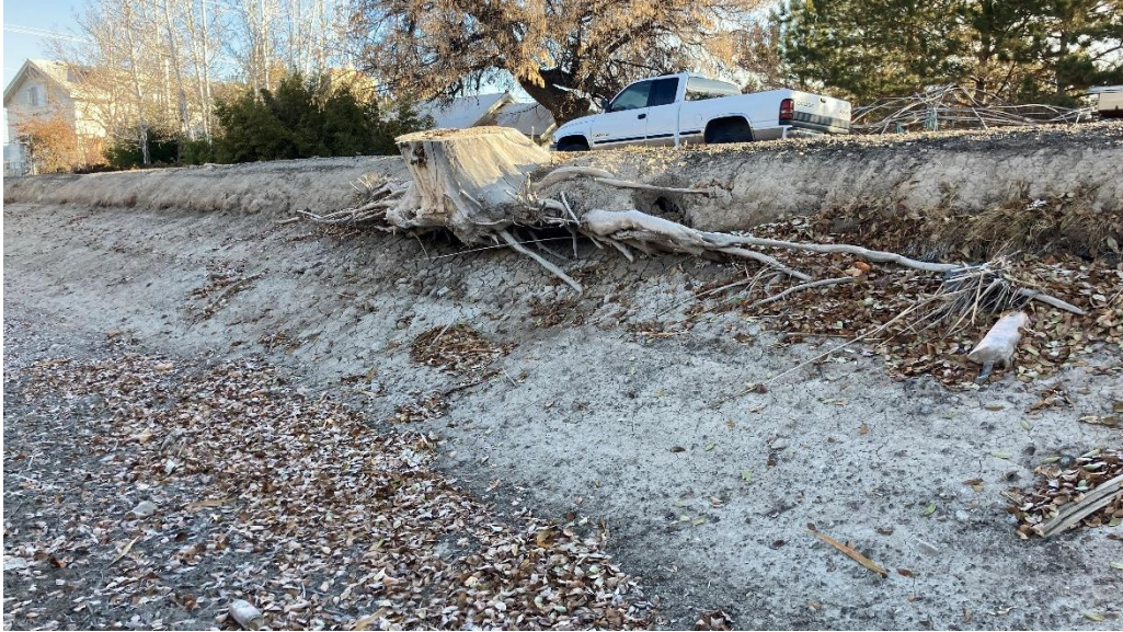
Photo 2-10: Tree Stump with Roots in the Utah and Salt Lake Canal Embankment
