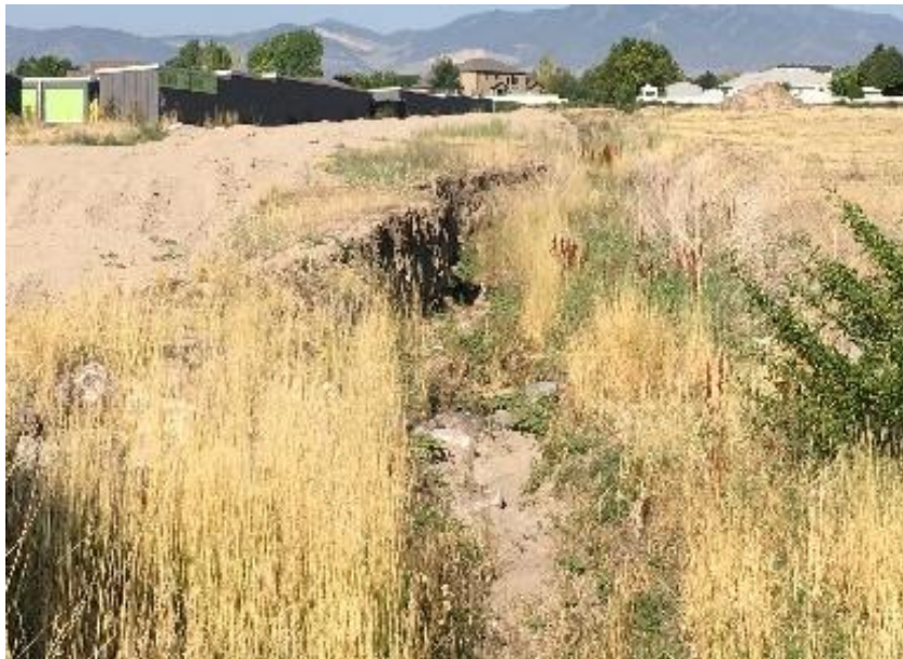
Photo 2-2: Bank Erosion Upstream of Airport Rd. on Barneys Creek
