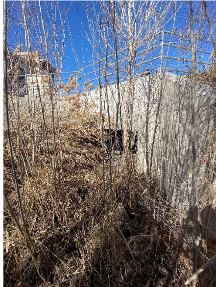
Photo 2-3: Excessive Vegetation in Channel on Bingham Creek near the Jordan Valley Medical Center
