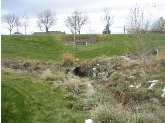
Upstream end of Rosecrest Road Culvert
