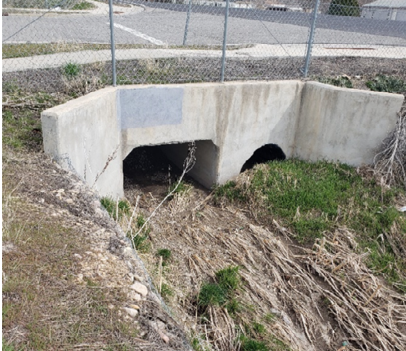
Downstream end of 13760 South Culvert
