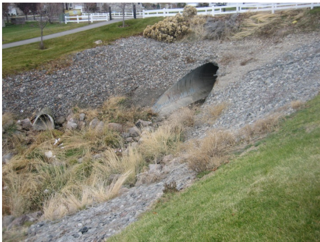
Upstream end of Friendship Drive Culvert
