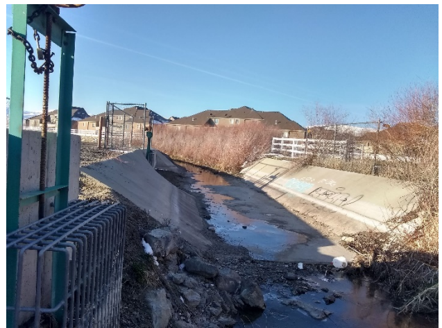
Utah Lake Distributing Canal
