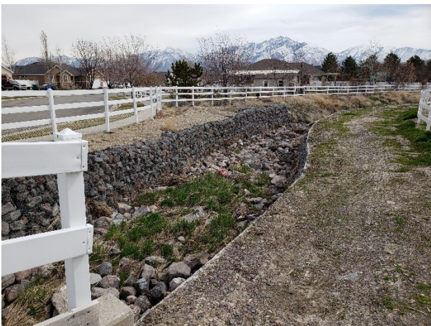
The channel downstream of the culvert at 3160 West
