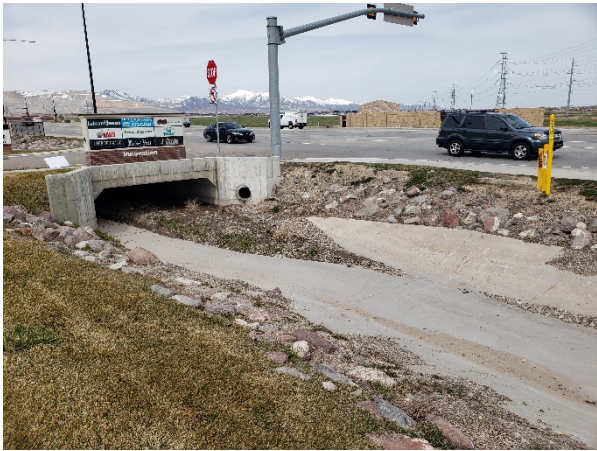
Downstream end of Millennial Lane Culvert
