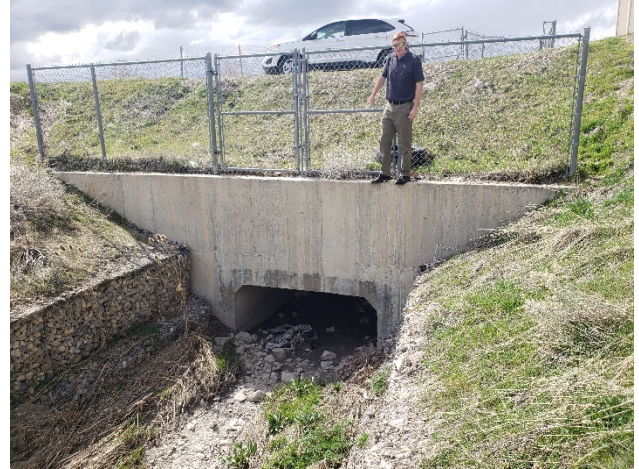
Downstream end of culvert crossing Utah and Salt Lake Canal
