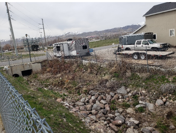
Rose Creek Channel upstream of the 13760 South Culvert
