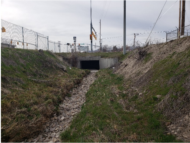
Upstream end of Bangerter Culvert
