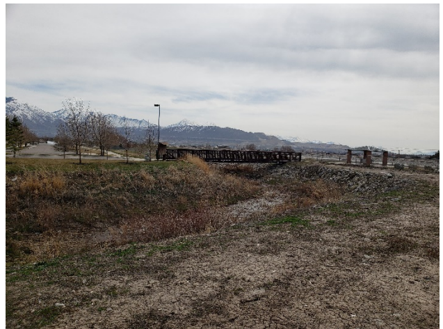
Footbridge at approximately 3350 West
