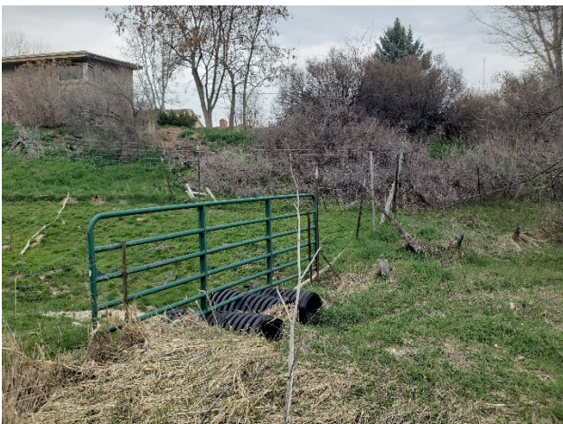
Fence crossing Rose Creek at approximately 1760 West
