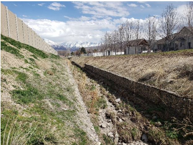
Rose Creek Channel Downstream of the Utah and Salt Lake Canal
