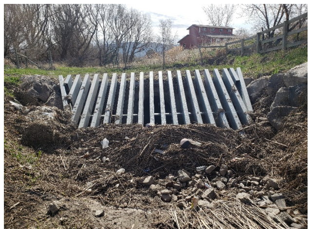
Trash Rack on 36-inch Pipe on Rose Creek at Approximately 2000 West
