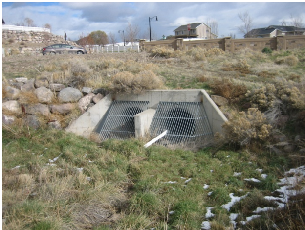
Upstream end of Mirabella Drive Culvert
