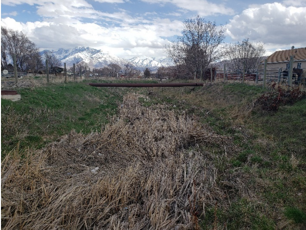
Pipe Crossing Rose Creek at 2150 West
