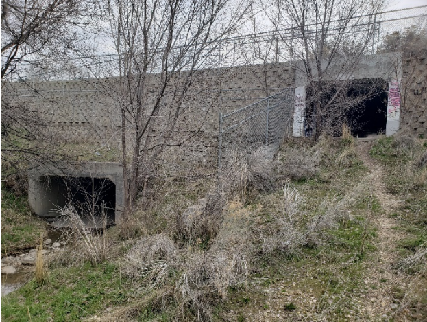
Upstream end Redwood Road Culvert
