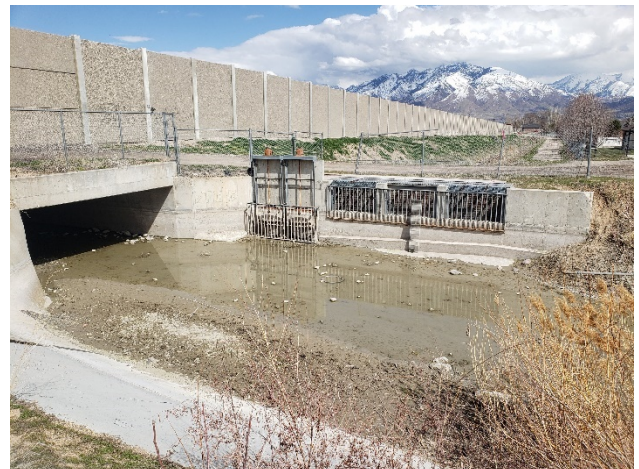
Utah and Salt Lake Canal Overflow Structure
