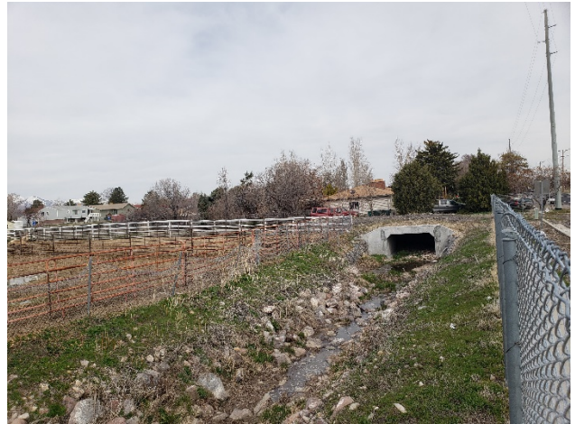
Downstream end of 90° Bend Culvert at 2700 West
