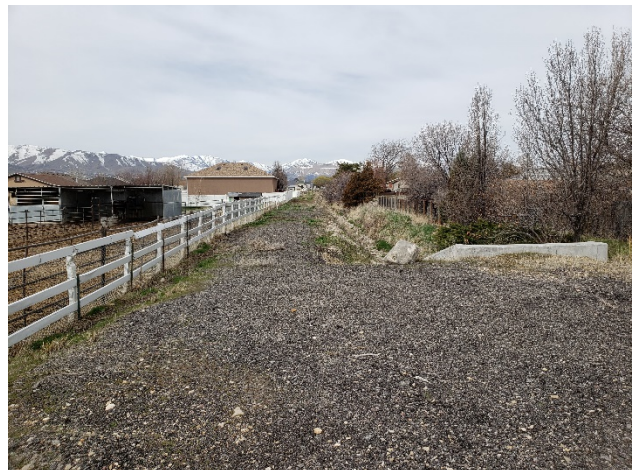
Rose Creek Channel Upstream of the 90° Bend Culvert at 2700 West
