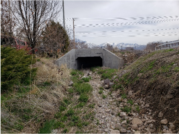
Upstream end of 90° Bend Culvert at 2700 West
