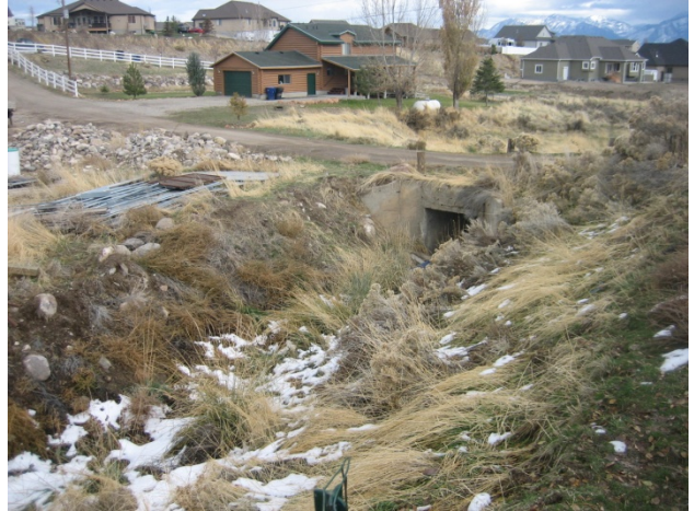
6100 West Culvert from Upstream
