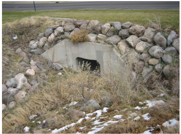
Upstream end of Spring Canyon Drive Culvert
