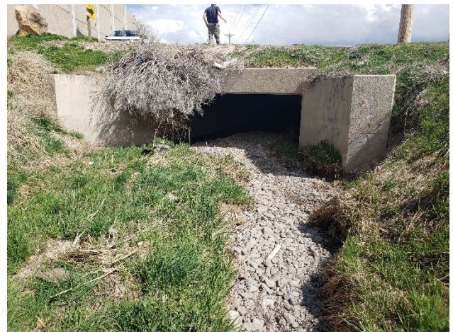
Upstream end of culvert crossing Utah and Salt Lake Canal
