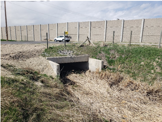
Downstream end of 2200 West Culvert
