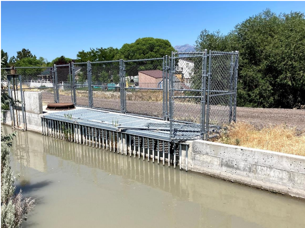
Photo 2-1 Overflow/Dump-Out Structure Where South Jordan Canal Crosses Midas Creek
