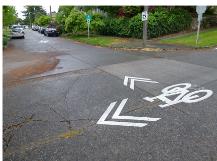
Example alternative pavement markings: SLMs with rotated chevrons. Note that these markings are not approved by FHWA. (Photo credit: Toole Design Group)
