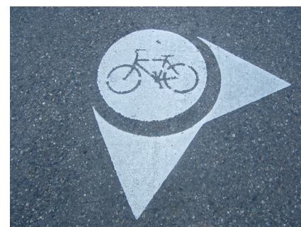
Example alternative pavement markings: "bike dots" (Photo credit: Toole Design Group)
