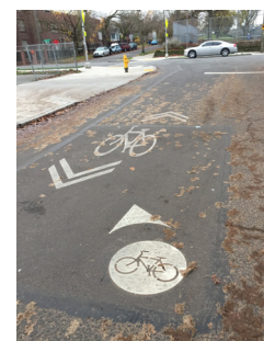
Application of bike dots (Photo credits: Toole Design Group)
