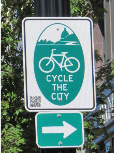
Local example of MUTCD M1-8a Bicycle Route sign for named route. Note that QR codes prohibited by MUTCD (Photo credit: Becka Roof)
