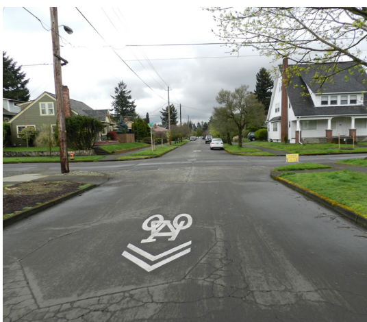
Standard application of SLMs for wayfinding (Photo credit: Toole Design Group)
