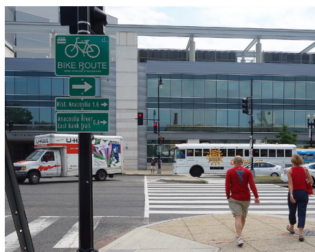
Example turn sign assembly (Photo credit: Toole Design Group)
