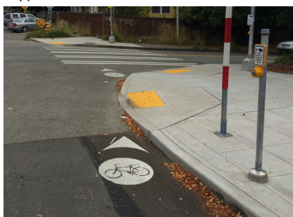
Application of bike dots (Photo credits: Toole Design Group)
