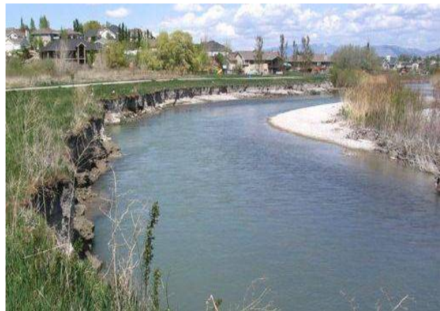
Figure 1.16 (above) and 1.17 (below). Example of a type F channel on the Jordan River in Riverton with shear eroding banks (above). The bank was graded back, rock placed along toe of bank to prevent erosion and planted with riparian vegetation (below) creating a type C channel.
