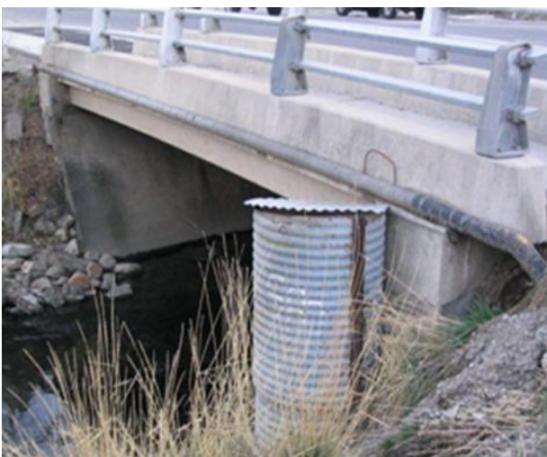
Figure 4.3 Stream flow gaging station on Big Cottonwood Creek.
