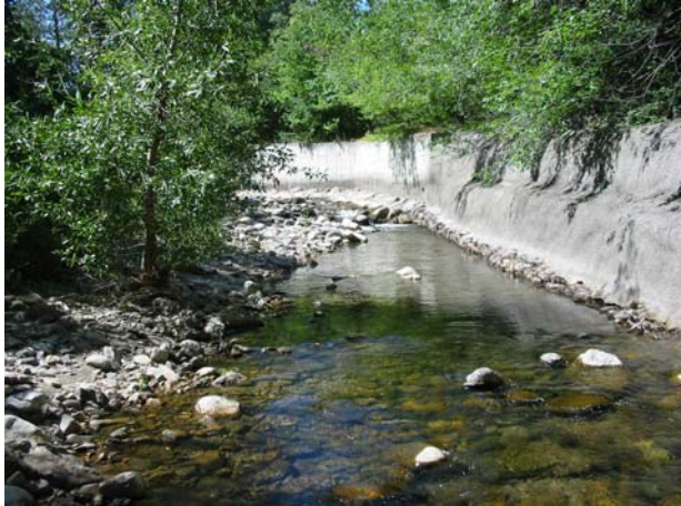
Figure 2.5 An example of bank stabilization that is counted as hydraulic alteration.
