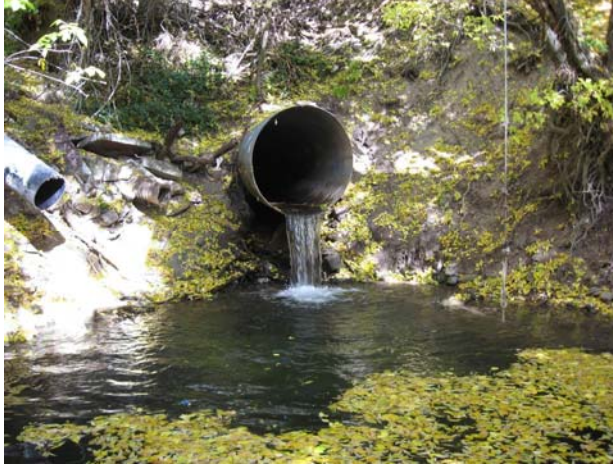
Figure 2.3 An example of a culvert that serves as a barrier to fish movement during the low flow season.
