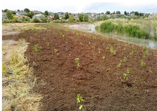
Figure 1.16 (above) and 1.17 (below). Example of a type F channel on the Jordan River in Riverton with shear eroding banks (above). The bank was graded back, rock placed along toe of bank to prevent erosion and planted with riparian vegetation (below) creating a type C channel.
