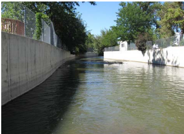
Figure 2.1 An example from Lower Big Cottonwood Creek that is channelized into a uniformly shallow streambed with no pool or riffle habitat diversity.
