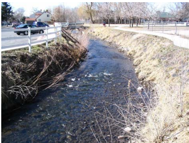
Mill Creek through Fitts Park in South Salt Lake.
