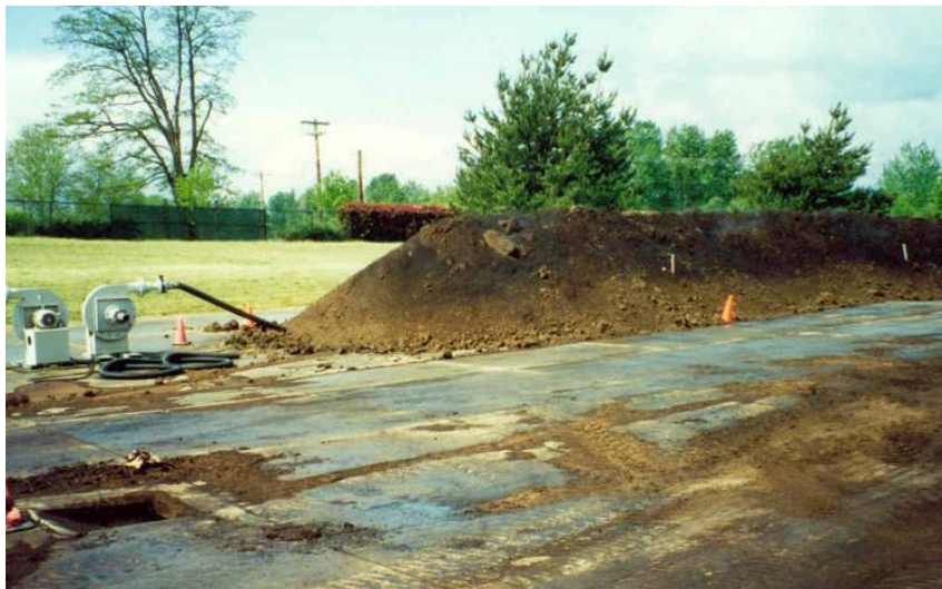
Figure 4-14 Example of Aerated Static Pile
