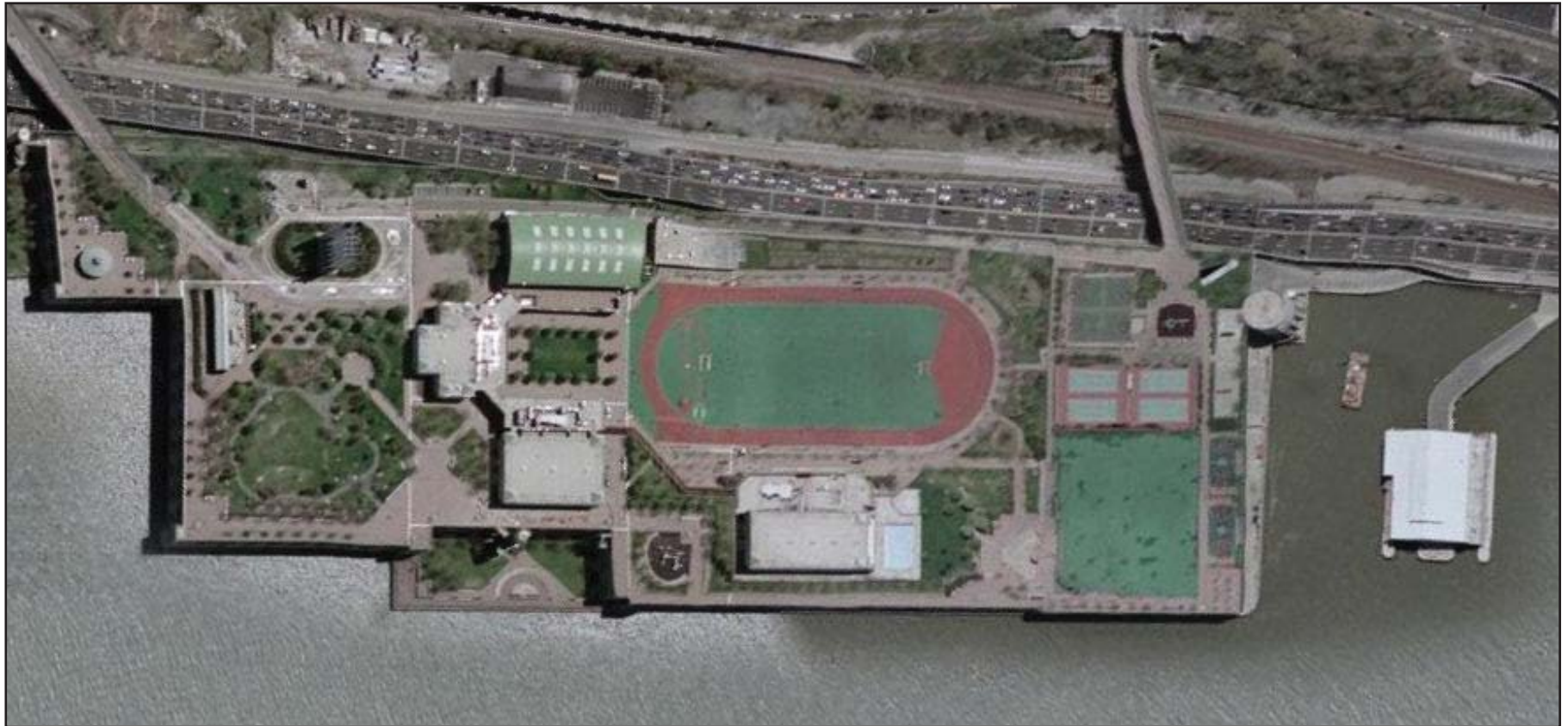
EXAMPLE OF A WWTP BENEATH A STATE PARK WITH COMMUNITY RECREATION FACILITIES ON THE SURFACE
