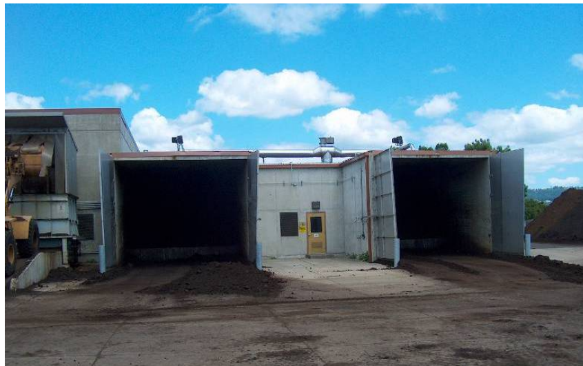
Figure 4-16 Example of In-Vessel System
