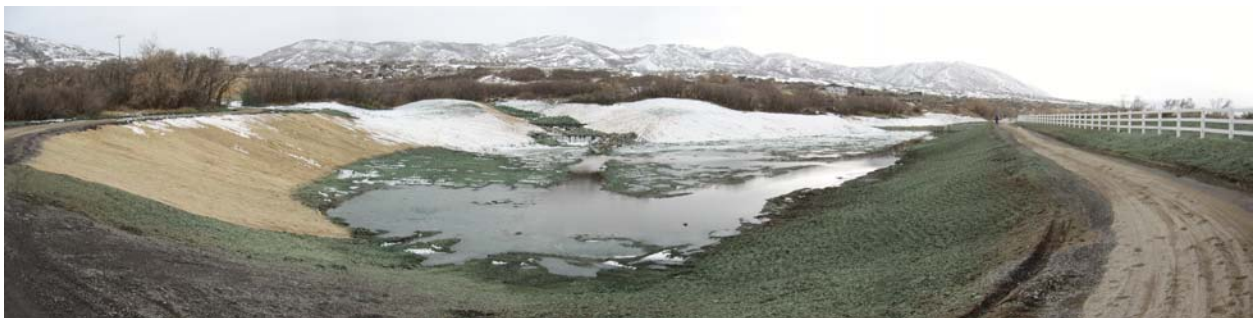
Corner Canyon Debris Basin, Lower Corner Canyon Sub-Watershed
