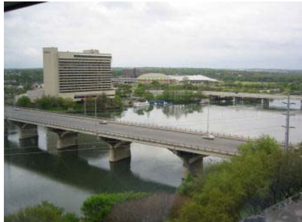
Example of urban/river interface, San Antonio River in Austin, TX
