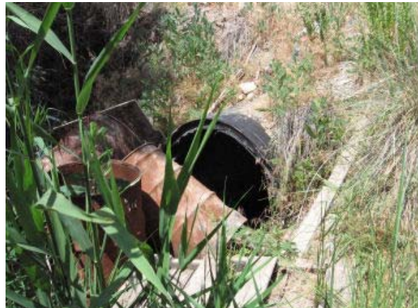
Harkers Creek Culvert, Coon/Harkers Sub-Watershed
