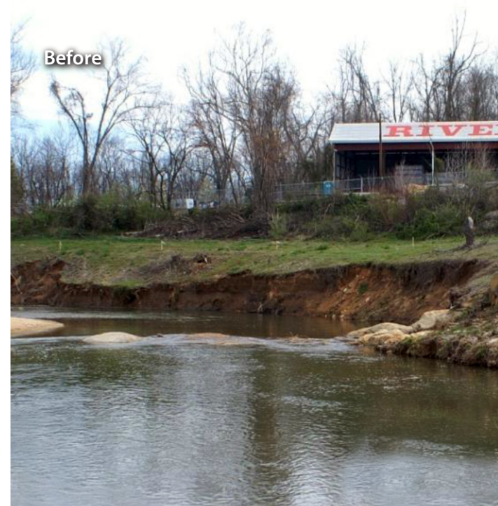
Bare and eroding banks are reshaped and revegetated in this stream restoration project that utilizes natural channel design techniques. (Photos: San Antonio River Authority)
