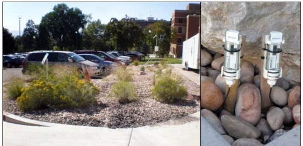
*What looks like a typical commercial landscape is actually a bioretention garden that collects and uses stormwater runoff at the University of Utah's Civil & Material Engineering building. Soil moisture meters (right) are used to monitor effectiveness, with the goal of installing bioretention gardens campus-wide.*
