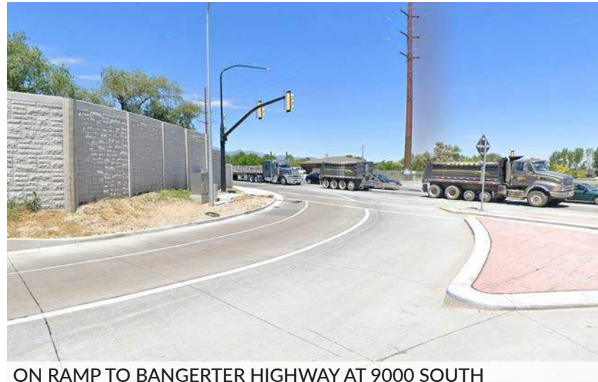
ON RAMP TO BANGERTEER HIGHWAY AT 9000 SOUTH
