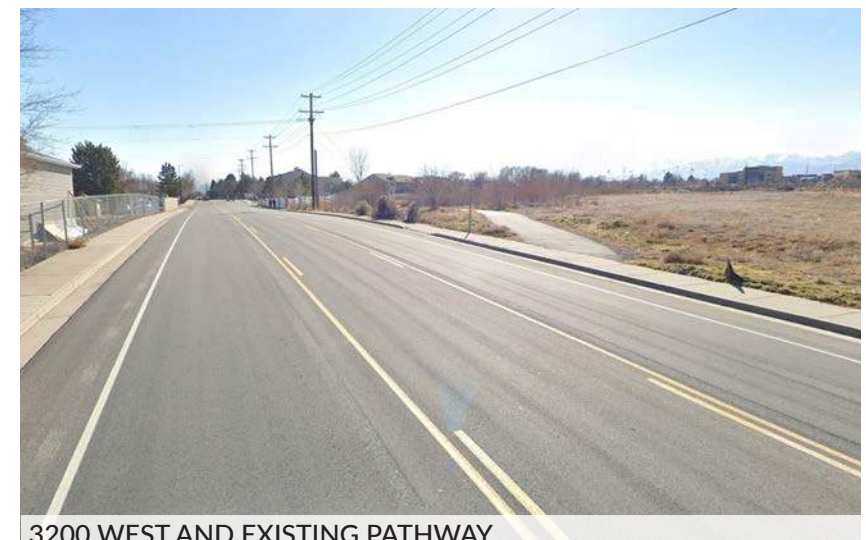
3200 WEST AND EXISTING PATHWAY
