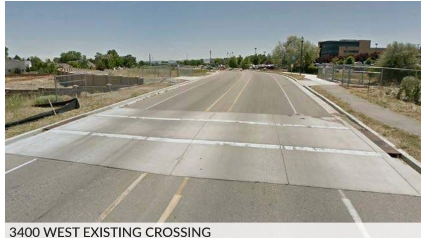
3400 WEST EXISTING CROSSING
