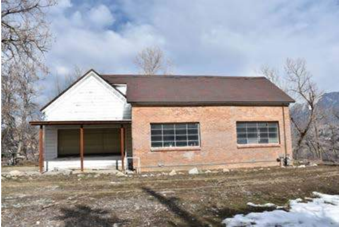
Photograph 3. Exterior, south elevations. Camera facing northeast.
