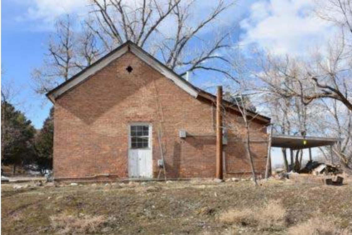
Photograph 5. Exterior, east elevation of east wing. Camera facing west.
