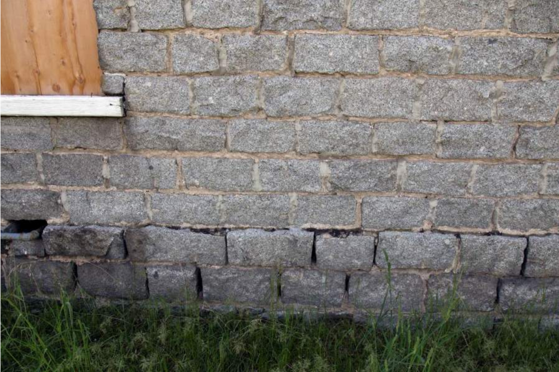
9 of 14. Granite brick foundation and wall detail. Camera facing south.
