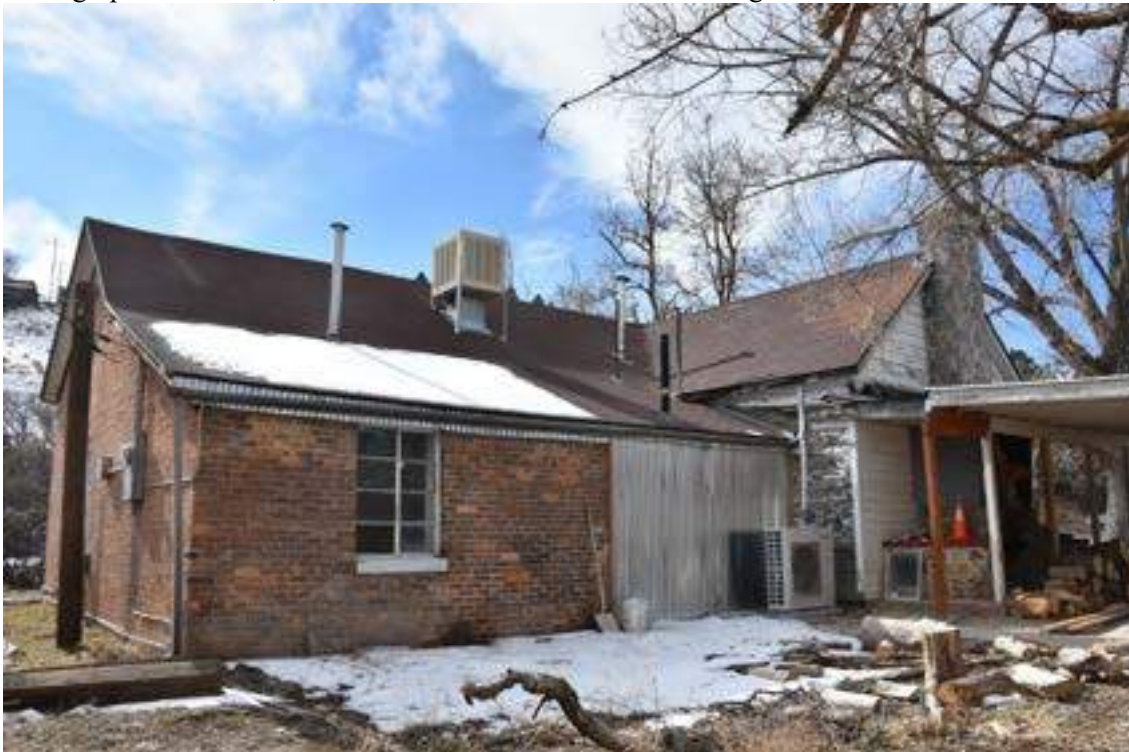
Photograph 6. Exterior, east and north elevations. Camera facing southwest.
