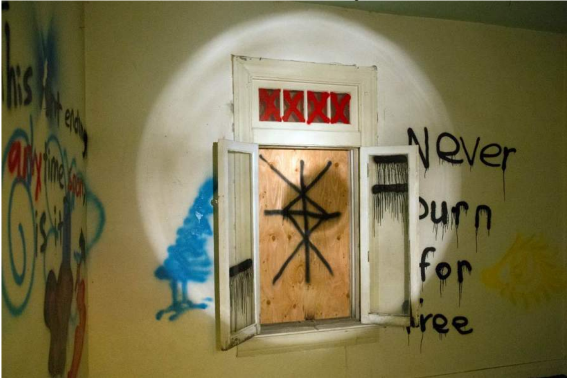
12 of 14. Interior window and wall detail. Camera facing north.
