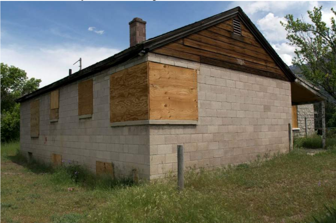
6 of 14. Southwest façade. Camera facing northeast.
