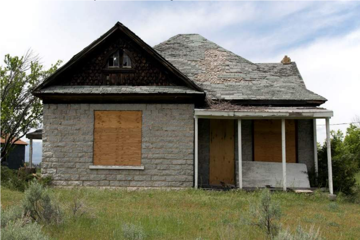
1 of 14. Front (east) façade. Camera facing west.
