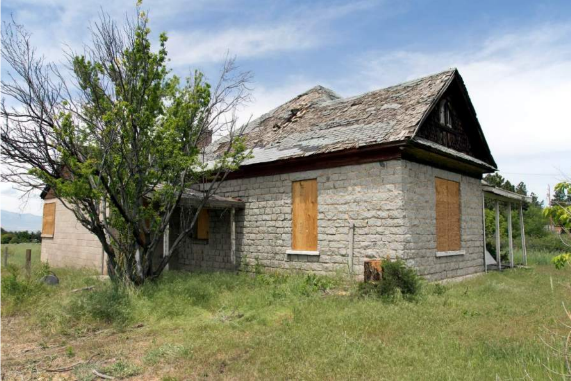
7 of 14. Southeast façade. Camera facing northwest.
