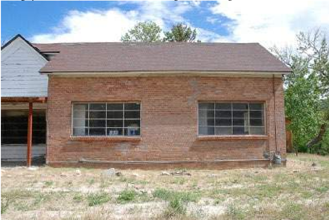
Photograph 4. Exterior, south elevation of east wing. Camera facing north.
