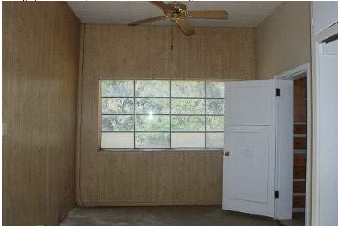
Photograph 13. Interior, east bedroom. Camera facing south.
