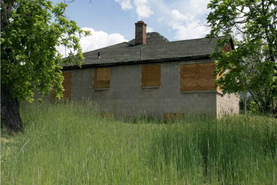
5 of 14. West façade. Camera facing east.
