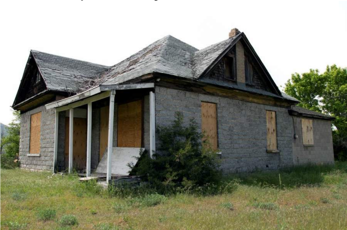
2 of 14. Northeast façade. Camera facing southwest.
