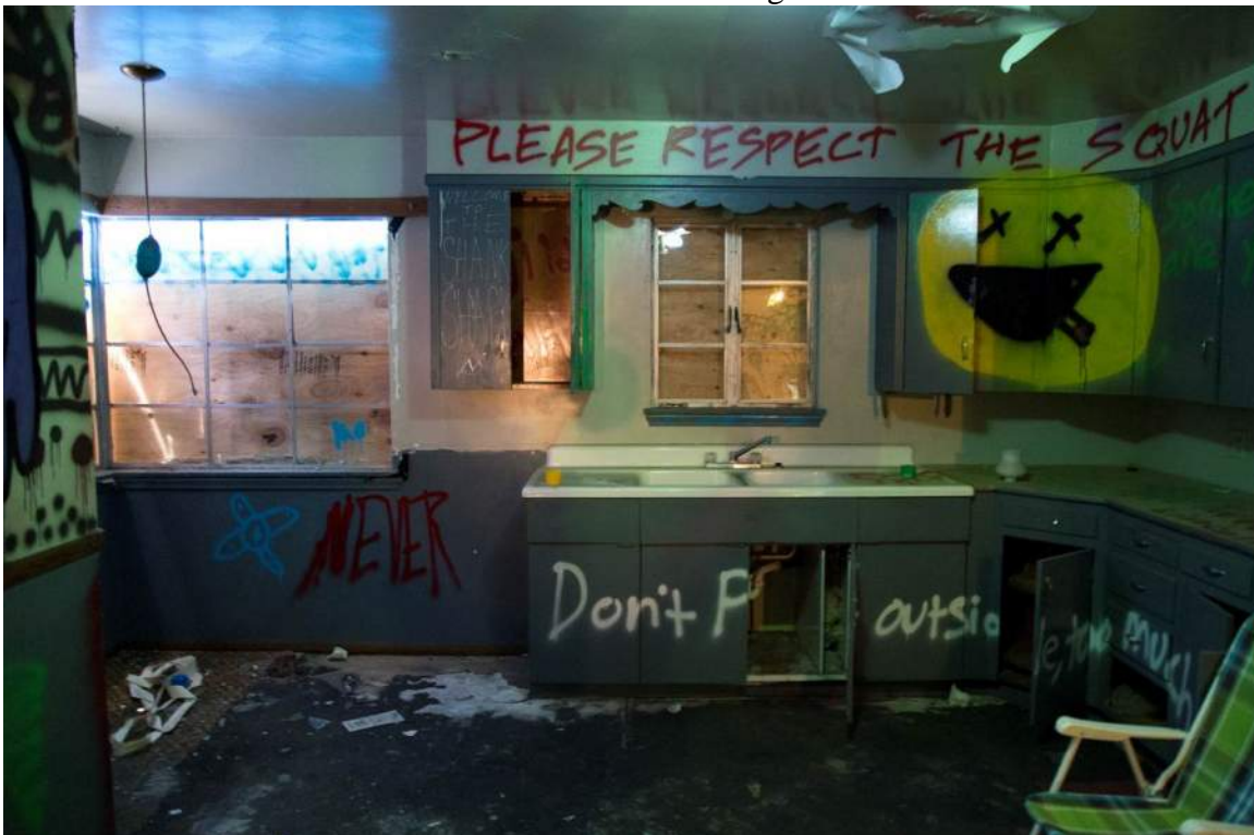
13 of 14. Interior kitchen addition detail. Camera facing west.
