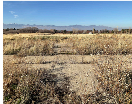
Remaining foundation of the barn
