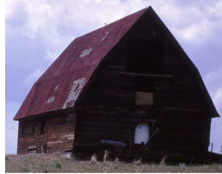
Original barn structure
