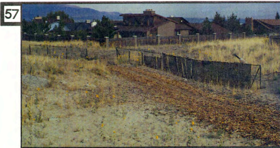
57 A) Until recently, residences living adjacent to the north rim of the Park, were bothered by the build up of drifting sand against their homes. This problem occurs primarily in the vicinity of the Salt Lake aqueduct and abandon sand pit areas. However, the problem does exist to a lesser degree, all along the north rim. Dispersing shredded woodchips on the surface of trails, has kept the sand from migrating into residential and other nearby areas.
