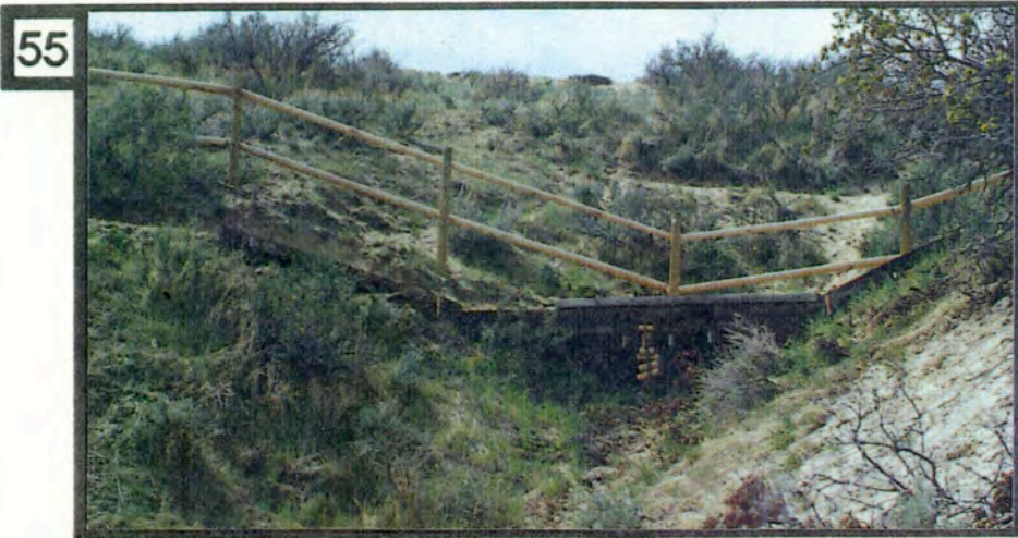
55 A) When a residential sub-division was developed west of this location, a log fence and retaining wall were constructed. The fence now serves to delineate the park boundary and discourage indiscriminate entry into the park. B) The retaining wall which supports the realigned trail, needs to be constructed better. When constructing any structures in the park, materials and construction techniques should have a long life expectancy.
