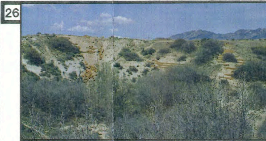
26 A) Using bales of straw to stabilize erosion should only be a temporary solution to a long term problem. Maintenance of the bale structures is necessary to extended the usefulness of this type of erosion mitigation. Stopping the drainage of water from entering the park from adjacent properties, will help prevent this type of damage.
