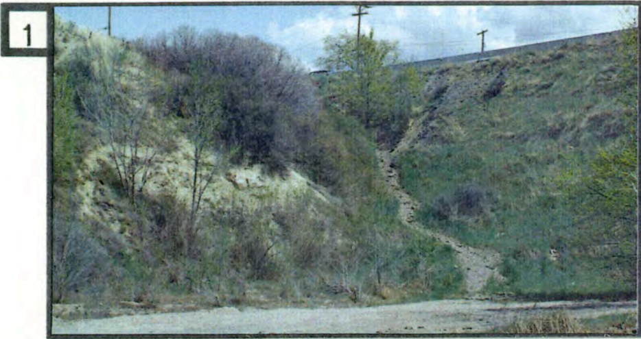
1 A) This area has been disturbed by user trails, brush fires and the construction of the 700 East roadway. Soil erosion has increased following each of these disturbances. B) The native trees and shrubs are water stressed from six years of drought conditions. C) Only annual grasses and noxious weeds are found growing on the steep embankment of the 700 East roadway.
