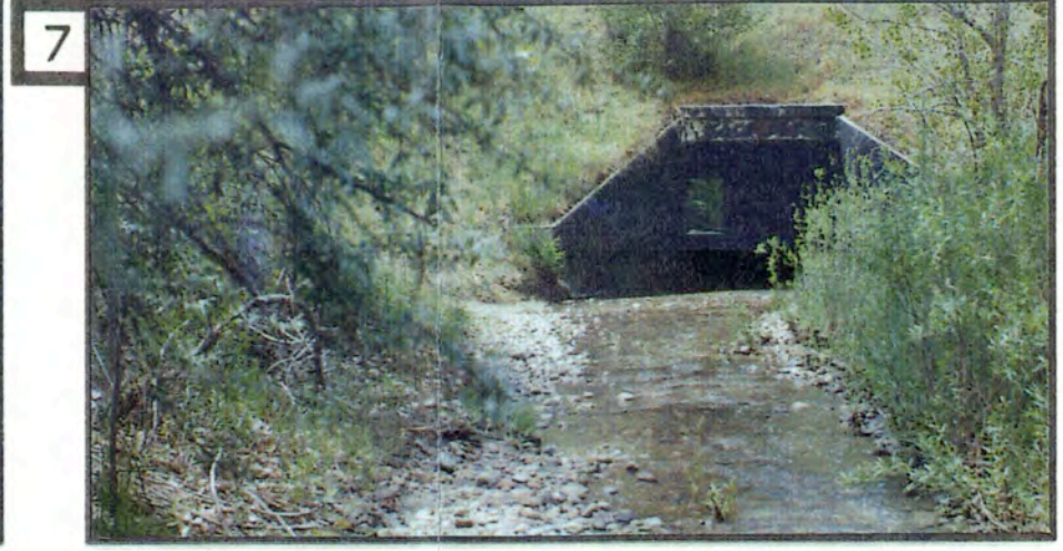
7 A) This section of Dry Creek is a good example of a stable streambed. Its strengths are: a healthy riparian community along the streambank, cobble rock lining of the streambed, and a stable water flow gradient. B) Stream "blow-out" at the outflow end of the culvert is a problem and prevents safe passage for trail users.
