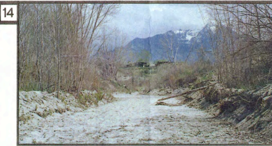
14 A) Maintaining a workable flow gradient in this section of Dry Creek is a constant effort for county flood control personnel. The erosion and deposition of adjacent streambanks into the streambed, is the cause of the problem. It is important to keep this section of Dry Creek flowing and minimize the amount of sediment transported through the culvert beneath the landfill. B) A high percentage of vegetation in this area is either stressed or strained.
