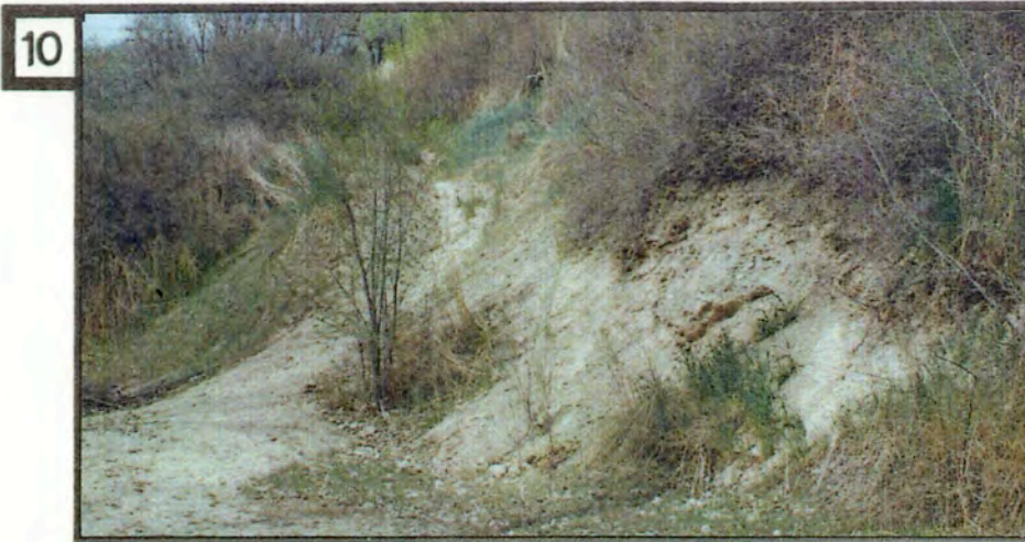
10 A) In areas of the park where high use is expected, measures need to be taken to prevent further loss of soil and vegetation. At this trail junction, the bottom of the slope is highly erodible and loose. Stabilizing this slope will insure that the trail will remain safe for use. B) Existing vegetation above the erosion scar will continue to slough down the slope until this erosion problem is stabilized.
