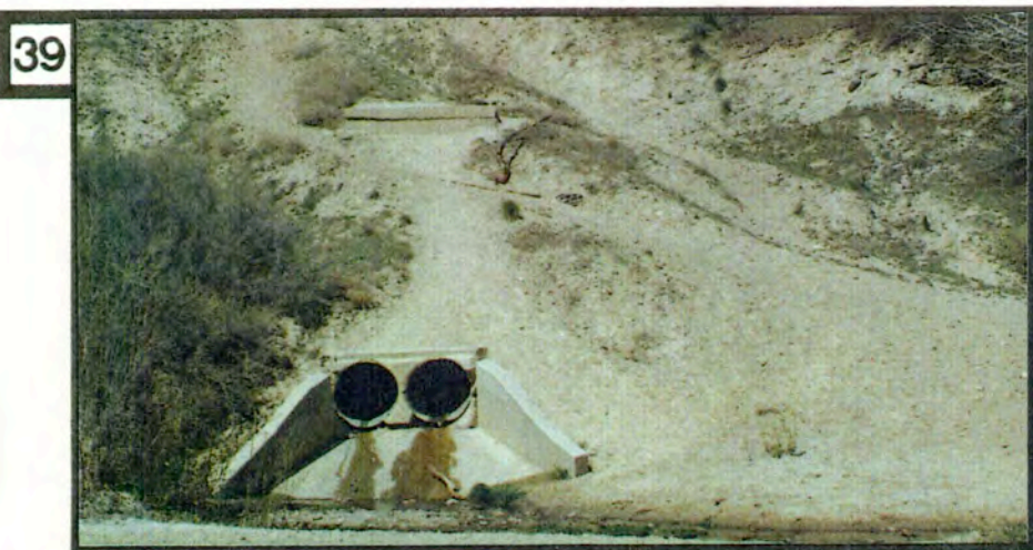
39 A) Trails aligned on top of utilities, perpetually erode soils into Dry Creek. Additionally, the barren ground associated with nearly all utility locations, remains without vegetation because of relentless trail usage. B) Because of splashing noises, most equestrian users are very cautious when riding past this particular outlet. Water spilling onto the concrete apron, startles most horses.
