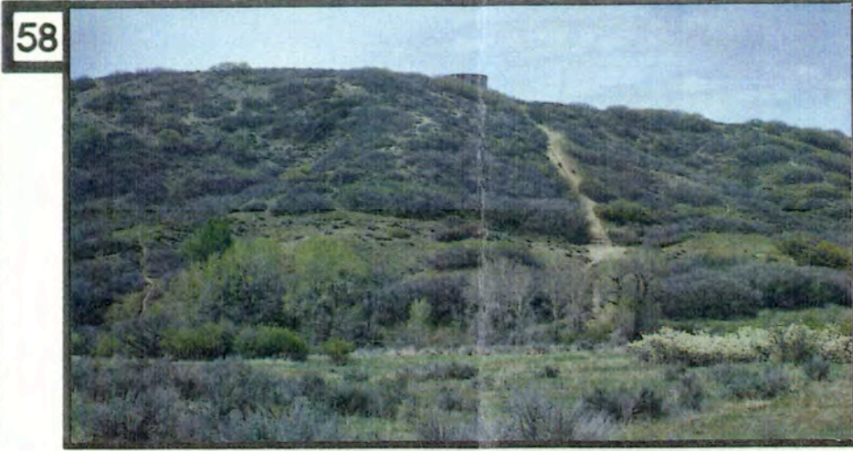
58 A) Utility installation scars are visible from several locations in the park. Many of these utility corridors have been used as trails for so many year, that native vegetation has never had a chance to recover and stabilize these disturbed areas.
