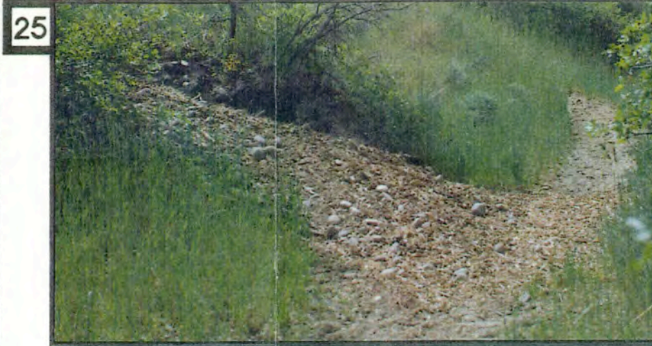
25 A) Before shredded bark chips were placed on this equestrian trail, soil erosion was out of control. Even though the slope continues to erode, erosion has slowed and the trail is safer for all park users. B) The placement of shredded wood chips on trails, serves to prevent trails from widening.
