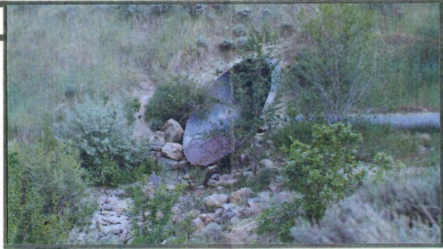
A) Stream flow velocities increase when passing through culverts. On the west side of the 1300 East road crossing, the streambed drops approximately two feet as it leaves the culvert. B) Trail conditions entering the culvert are awkward and dangerous because of the number of large boulders and elevation change.
