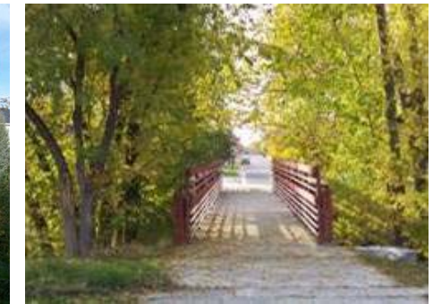
Figure 3.10.53 Bridge B24 7' wide, 77' span, 6' clearance
