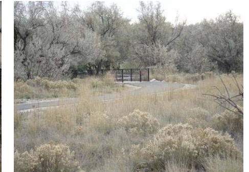
Figure 3.2.11 Footbridge along Spring View Farms Trail
