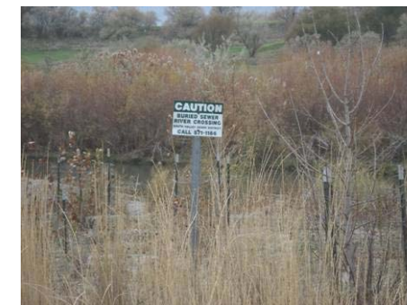
Figure 3.3.13 Buried sewer river crossing sign west of trail
