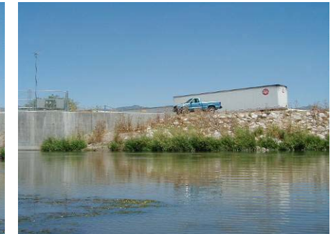
Figure 4.9.10 Surplus dam, gravel with no path (WP 10-14)
