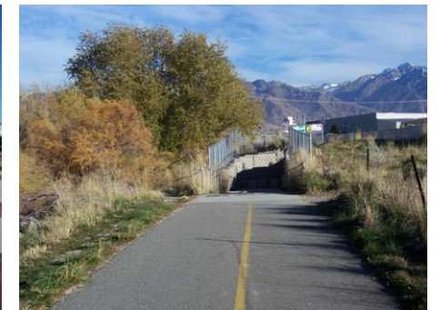
Figure 3.8.13 4700 South pedestrian underpass
