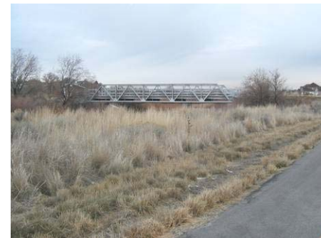
Figure 3.3.29 Bridge B4 24' wide, 73' span, 12' clearance
