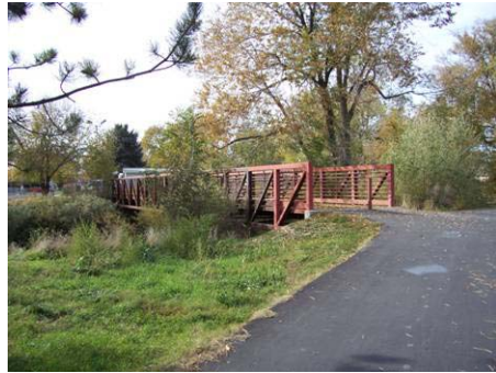
Figure 3.10.37 Bridge B21 10' wide, 100' span, 6' clearance
