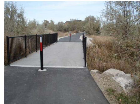
Figure 3.2.6 Footbridge along Jordan River Trail
