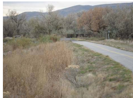
Figure 3.2.20 View looking south at footbridge (Figure 2.19)
