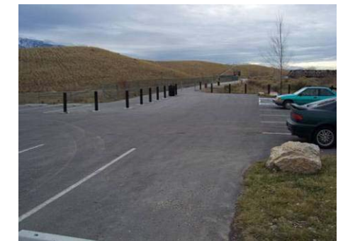
Figure 3.6.12 Midvale Center Street Trailhead parking lot
