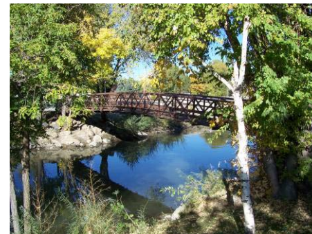
Figure 3.11.3 Bridge B25 6' wide, 75' span, 9' clearance
