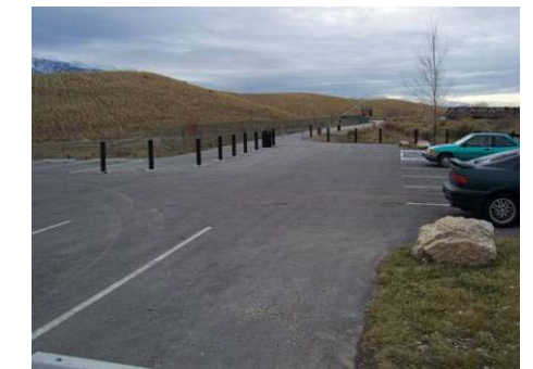
Figure 3.6.12 Midvale Center Street Trailhead parking lot
