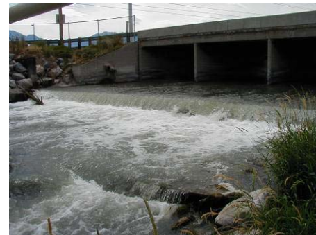
Figure 4.7.2 Pipeline, bridge at 6400 South (WP 9-02)
