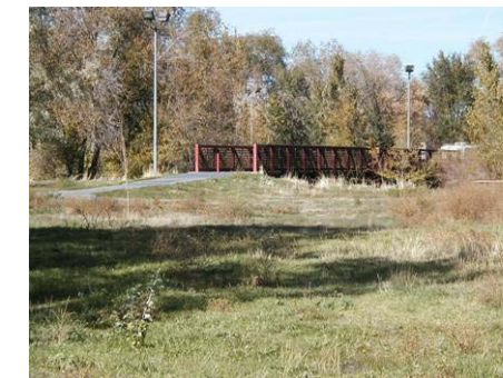
Figure 3.10.32 Bridge B20 10' wide, 100' span, 6' clearance
