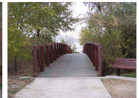
Figure 3.9.14 Bridge B15 10' wide, 120' span, 15' clearance
