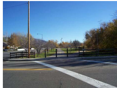
Figure 3.7.22 At-grade crossing, north of Cottonwood Grove Park
