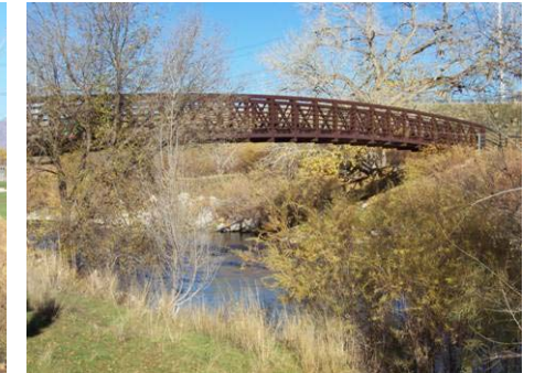
Figure 3.7.11 Bridge B9 6' wide, 120' span, 16' clearance
