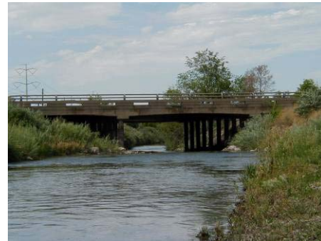
Figure 4.6.4 Vehicular bridge at 7800 South (WP 8-05)
