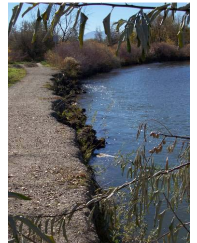
Figure 5.6.2 Section of Trail Washed Out
