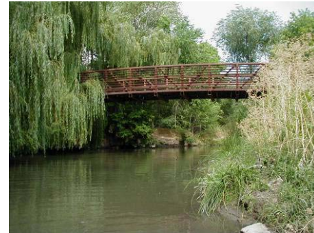
Figure 4.10.14 High footbridge (WP 11-26)
