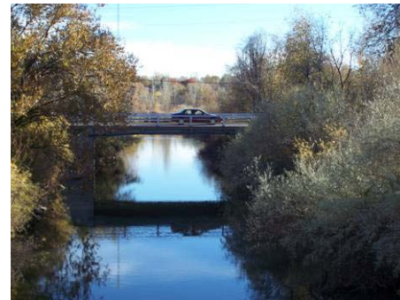
Figure 3.8.7 View to south from Bridge B13
