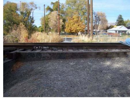
Figure 3.10.43 Non-accessible railroad crossing south of 900 South
