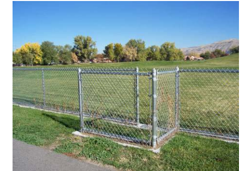
Figure 5.3.6 Trail Access Point
