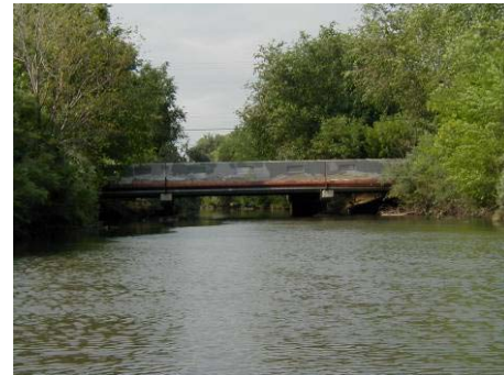
Figure 4.10.16 Low bridge at 500 South (WP 11-29)
