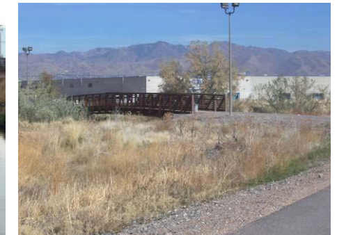
Figure 3.9.59 Bridge B17, 10' wide, 100' span, 8' clearance
