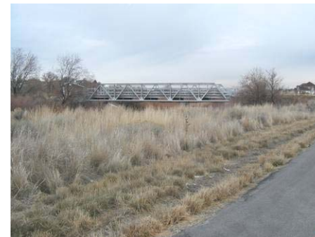
Figure 3.3.29 Bridge B4 24' wide, 73' span, 12' clearance
