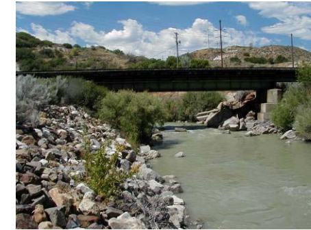
Figure 4.1.4 Portage put-in for the Turner Dam at the Narrows (WP 3-03)
