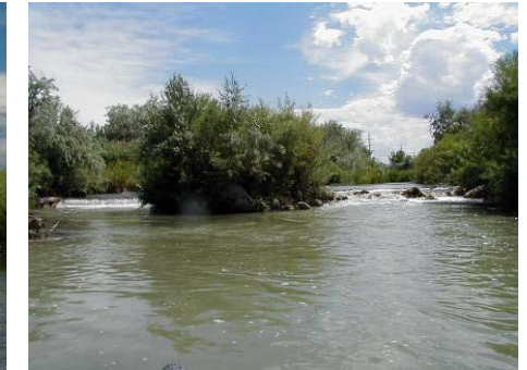
Figure 4.5.11 Waterfall created by sewer pipe (WP 8-01A)
