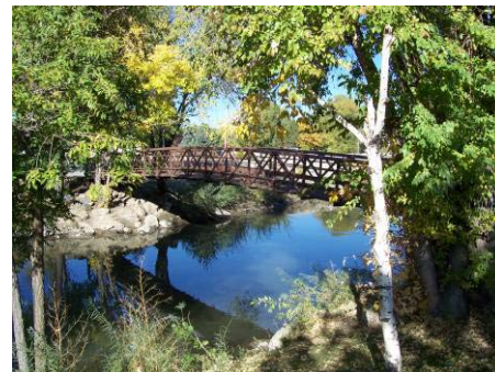
Figure 3.11.3 Bridge B25 6' wide, 75' span, 9' clearance
