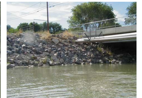
Figure 4.2.14 Questar Pipeline upstream of bridge (WP 4-32)
