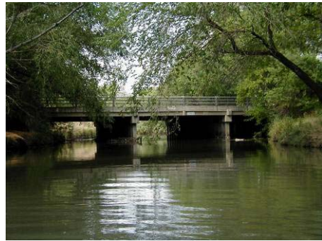
Figure 4.10.15 Vehicular bridge at 700 South (WP 11-27)
