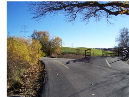
Figure 3.7.14 View toward neighborhood access east of Bridge B9
