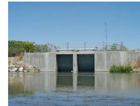
Figure 4.9.9 Diversion dam for surplus canal at 2100 South (WP 10-13)
