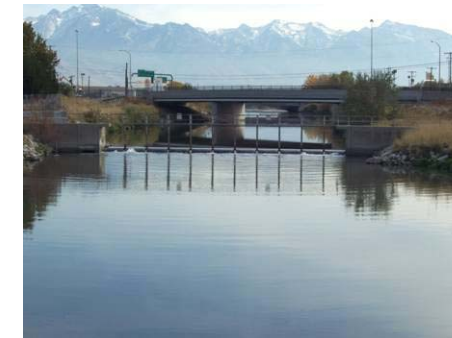
Figure 3.9.58 View from footbridge toward diversion dam and 2100 South overpass
