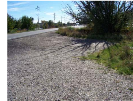
Figure 3.12.12 Informal parking west of Redwood Road
