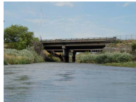
Figure 4.7.7 Vehicular bridge at Interstate 215 (WP 9-08)
