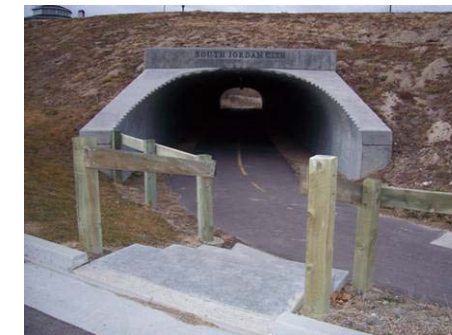
Figure 3.5.12 Shield's Lane pedestrian underpass
