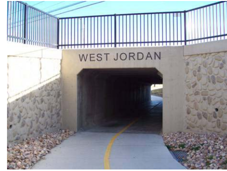
Figure 3.6.50 Winchester Street underpass
