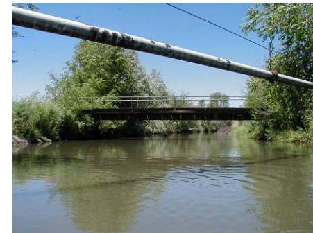
Figure 4.12.8 Footbridge, pipeline near Redwood Road (WP 14-02)
