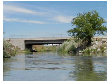
Figure 4.4.7 Bridge at 10600 South, potential launch site (WP 6-17)
