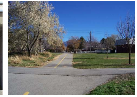
Figure 3.7.35 Germania Park Trailhead, north of 5400 South
