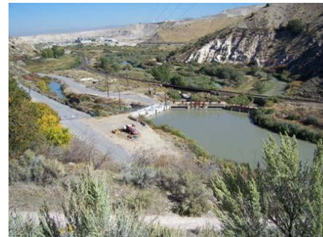
Figure 3.1.3 View to northwest, overlooking Jordan Narrows Diversion Dam and Canals
