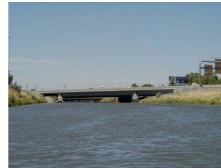
Figure 4.9.4 Bridge at SR-201 (WP 10-10)
