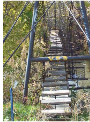
Figure 3.12.28 Structure spanning river
