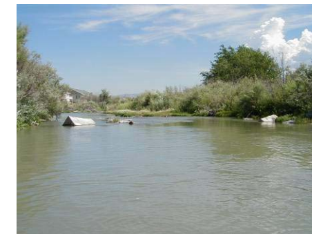
Figure 4.3.15 Concrete riprap in channel, boulders, debris (WP 6-08)
