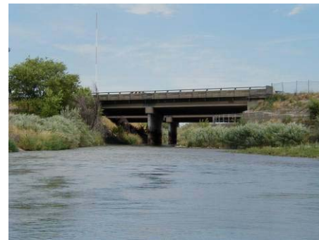
Figure 4.7.7 Vehicular bridge at Interstate 215 (WP 9-08)
