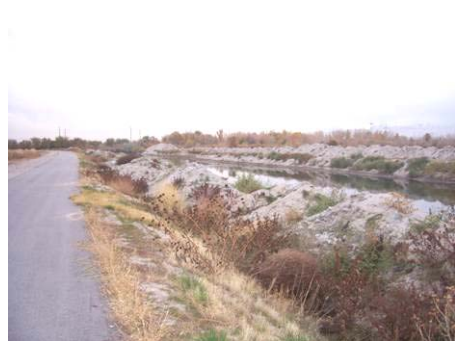
Figure 3.9.19 Dredging piles along Jordan River near Redwood Nature Area
