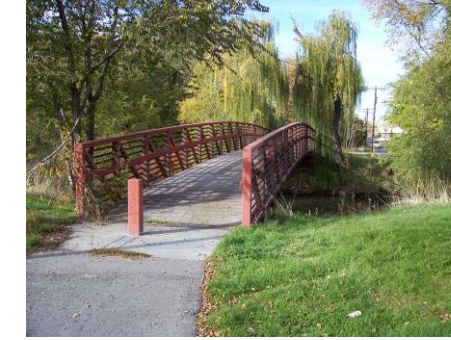
Figure 3.10.50 Bridge B23 10' wide, 100' span, 11' clearance
