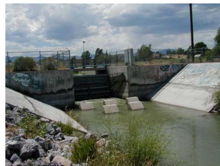
Figure 4.5.6 Irrigation dam at 9600 South (WP 7-08)
