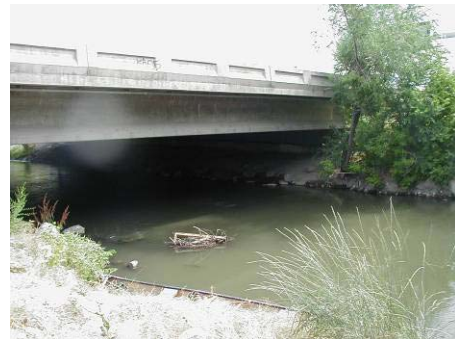
Figure 4.11.1 Interstate 80 Bridge (WP 12-03)
