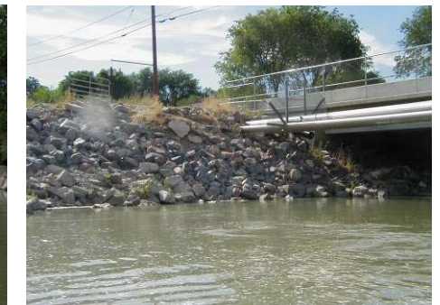
Figure 4.2.14 Questar Pipeline upstream of bridge (WP 4-32)
