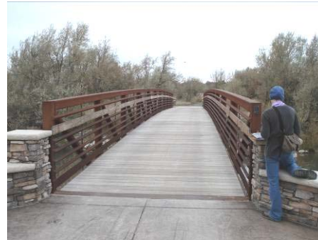
Figure 3.2.2 Bridge B1 10' wide, 100' span, 6' clearance
