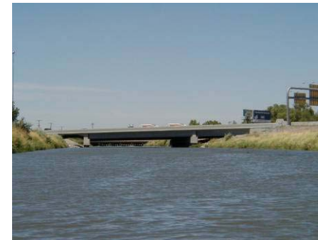
Figure 4.9.4 Bridge at SR-201 (WP 10-10)
