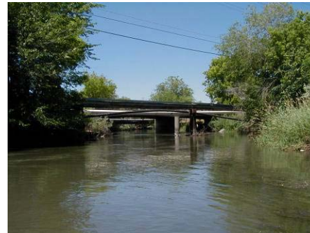
Figure 4.12.5 Pipeline across river (WP 13-07)
