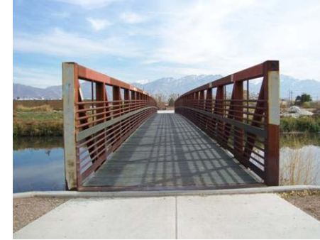
Figure 3.9.48 Bridge B16, 10' wide, 165' span, 11' clearance
