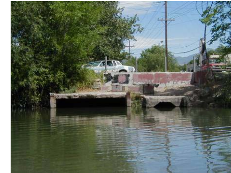
Figure 4.10.5 Storm drain, tributary at 1200 South (WP 11-15)
