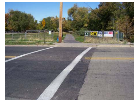
Figure 3.11.27 Crosswalk at 500 North
