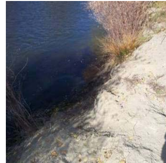
Figure 3.7.42 Washed out trail edge, west of Germania Park
