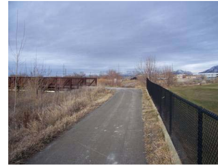
Figure 3.5.26 Bridge B7 10' wide, 130' span, 8' clearance
