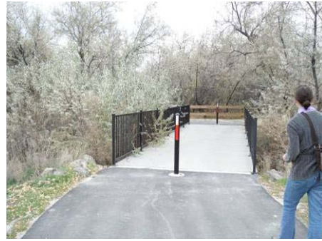
Figure 3.2.19 Footbridge south of Bangerter Highway
