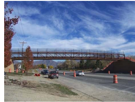
Figure 3.8.21 3900 South pedestrian sky bridge
