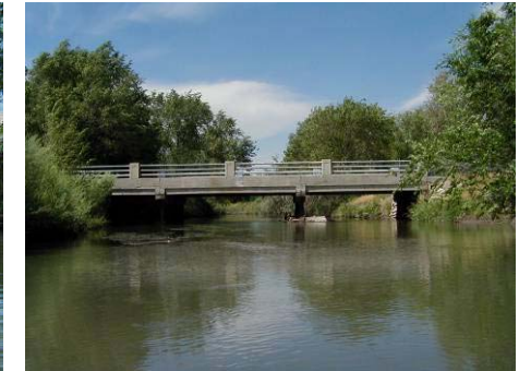
Figure 4.10.6 Bridge at California Avenue (WP 11-16)
