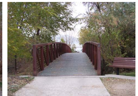
Figure 3.9.14 Bridge B15 10' wide, 120' span, 15' clearance
