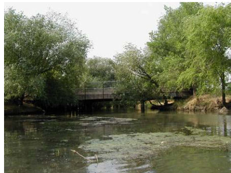
Figure 3.10.17 Vehicular bridge at 400 South (WP 11-30)
