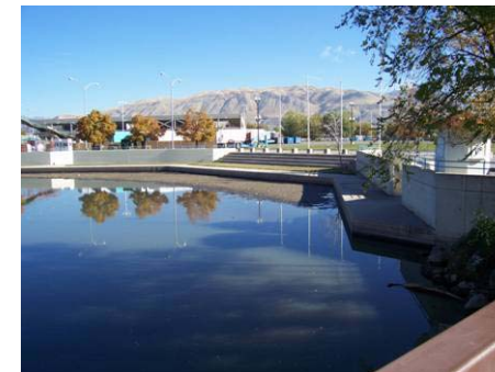
Figure 3.11.4 View from Bridge B25 towards Utah State Fair Park
