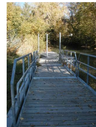
Figure 3.10.28 Boat ramp in Neighborhood Park
