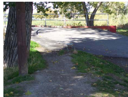
Figure 3.12.3 Bridge B31 12' wide, 54' span, 6' clearance
