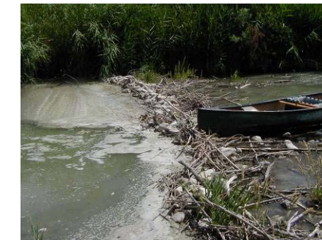
Figure 4.2.11 Rock weir (WP 4-21)
