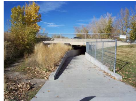
Figure 3.9.2 3500 South pedestrian underpass, looking north
