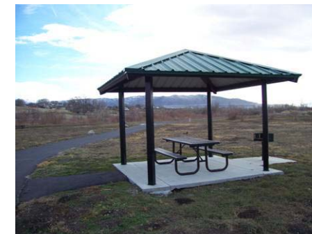
Figure 3.4.12 Picnic pavilion along trail
