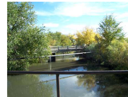
Figure 3.12.18 View to Redwood Road overpass from Bridge B32
