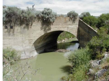
Figure 4.1.25 Railroad bridge at Lower Narrows (WP 4-01)
