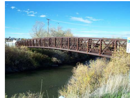
Figure 3.7.30 Bridge B10, 6' wide, 121' span, 15' clearance
