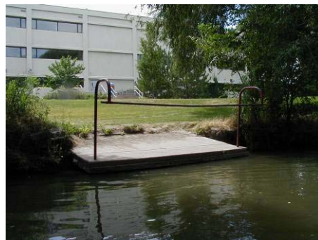
Figure 4.11.18 Concrete boat launch at Agriculture Building (WP 12-29)
