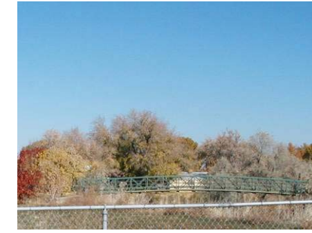
Figure 3.10.8 Bridge B18 4' wide, 69' span, 10' clearance
