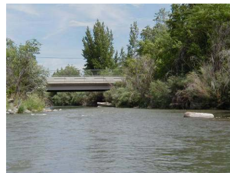
Figure 4.7.9 Vehicular bridge at Bouillon Street (WP 9-10)
