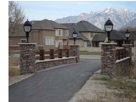
Figure 3.2.12 Footbridge along Jordan River Trail
