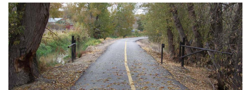
Figure 5.3.5 Trail Entry Barriers
