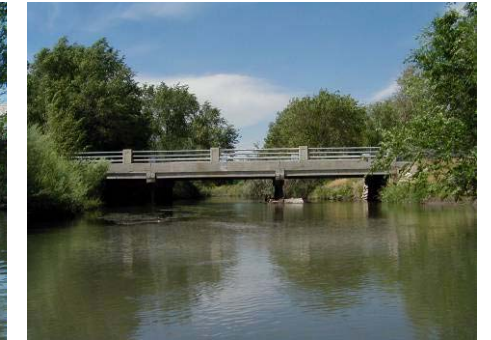
Figure 4.10.6 Bridge at California Avenue (WP 11-16)
