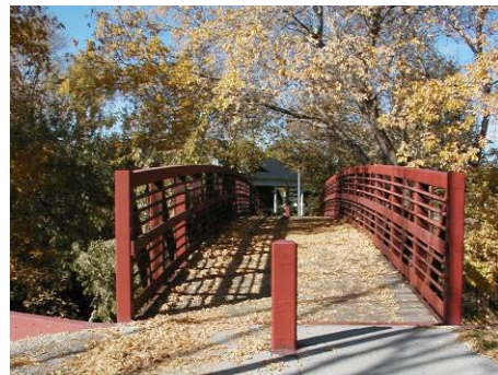
Figure 3.10.18 Bridge B19 10' wide, 100' span, 11' clearance
