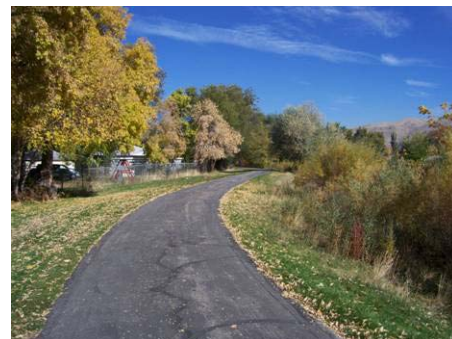
Figure 3.11.26 Trail north of Cottonwood Park, looking north
