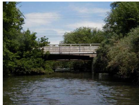
Figure 4.11.14 Overhead pipeline and cable at North Temple (WP 12-17)
