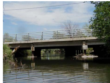
Figure 4.11.21 Bridge at 700 North, low clearance (WP 12-34)
