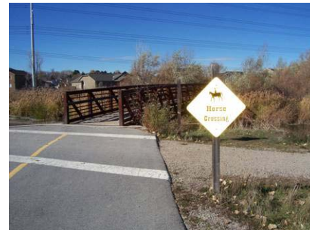
Figure 3.7.50 Bridge B12 8' wide, 122' span, 8' clearance
