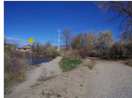
Figure 3.7.46 Re-routed equestrian trail, washed out
