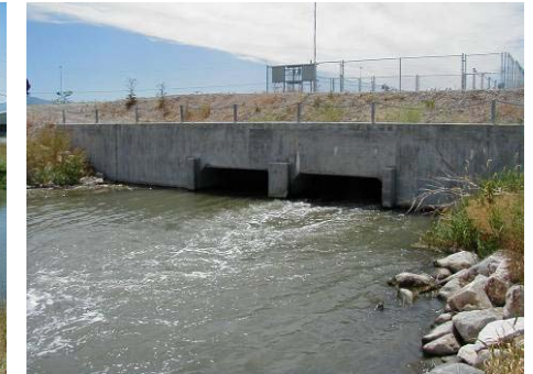
Figure 4.9.8 Diversion dam at 2100 South downstream (WP 10-13)
