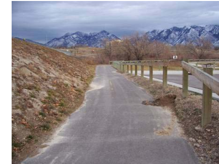
Figure 3.5.10 Trail looking east near 10000 South
