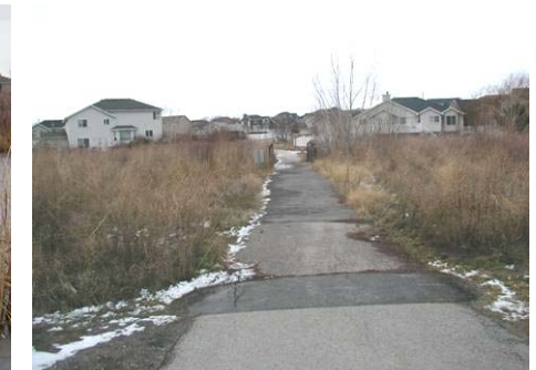
Figure 3.3.37 Paved access to neighborhood
