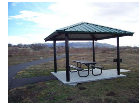
Figure 3.4.12 Picnic pavilion along trail
