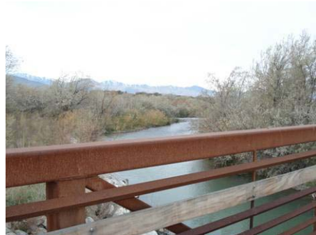
Figure 3.2.18 View to southeast from Bridge B1
