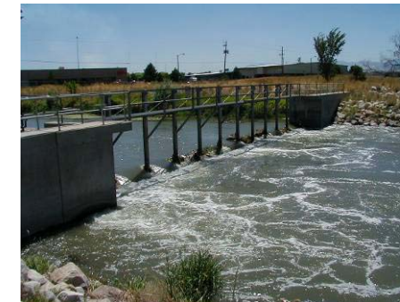
Figure 4.9.11 Weir at surplus canal at 2100 South (WP 10-16)
