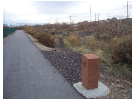
Figure 3.6.5 Crushed asphalt pathway
