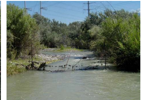
Figure 4.2.10 Barbed fence, river splits (WP 4-20)
