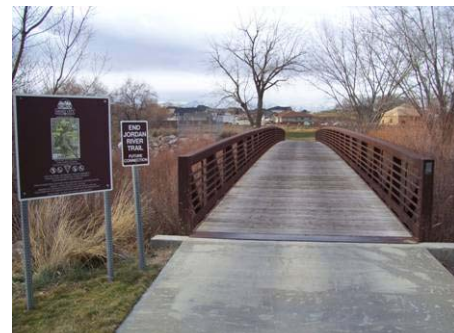
Figure 3.5.24 Bridge B5 10' wide, 130' span, 9' clearance
