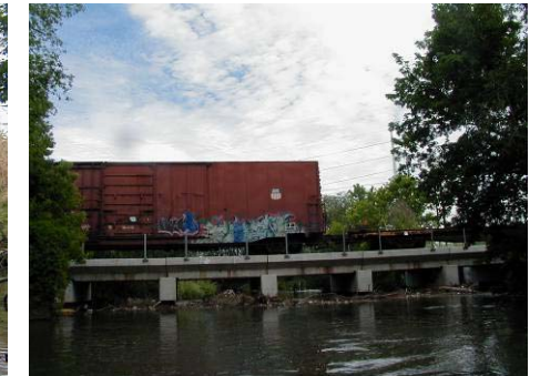
Figure 4.11.6 Concrete railroad bridge (WP 12-08)
