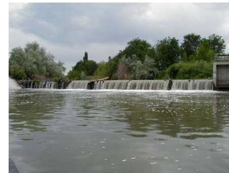
Figure 4.8.4 Weir at 4600 South (WP 9-23)
