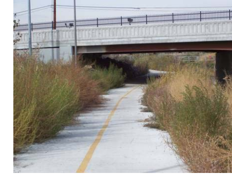
Figure 3.9.54 Pedestrian underpass, 2100 South, looking north
