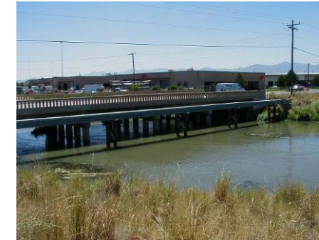
Figure 4.9.7 Pipeline across river near 2100 South (WP 10-12)
