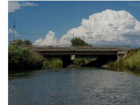
Figure 4.5.10 Vehicular bridge at 9000 South (WP 7-12)
