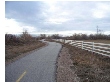
Figure 3.6.35 View from trail, looking south
