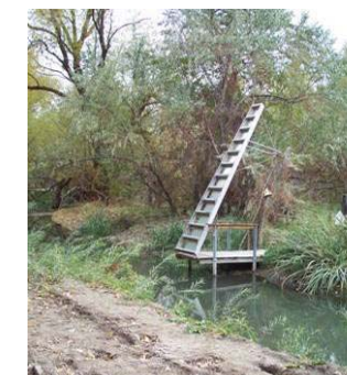
Figure 3.9.38 Drop-down bridge crossing canal in Redwood Nature Area
