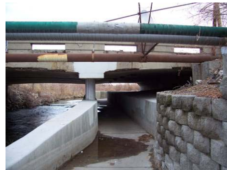
Figure 3.6.20 7800 South underpass, north side
