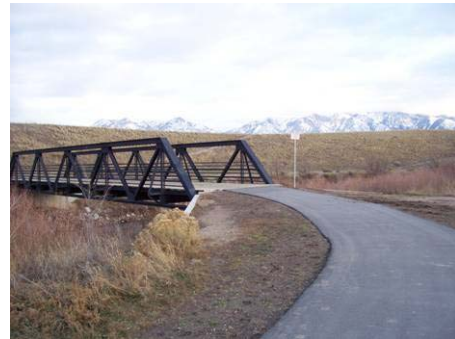
Figure 3.6.1 Bridge B8 16' wide, 90' span, 15' clearance
