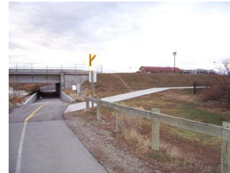
Figure 3.4.30 Trail connection to 10600 South near Mulligan's Golf
