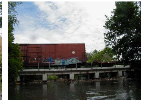
Figure 4.11.6 Concrete railroad bridge (WP 12-08)
