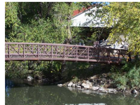
Figure 3.11.8 Bridge B26 8' wide, 77' span, 9' clearance
