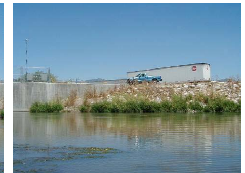
Figure 4.9.10 Surplus dam, gravel with no path (WP 10-14)
