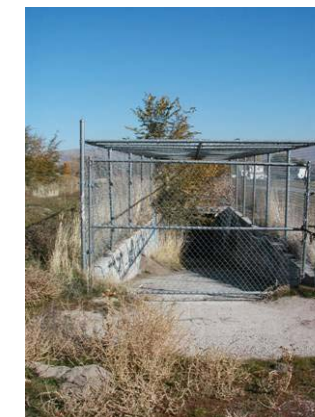
Figure 3.10.12 Utility Structure near informal Labyrinth path
