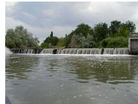
Figure 4.8.4 Weir at 4600 South (WP 9-23)
