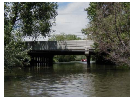
Figure 4.10.2 Vehicular bridge at 1700 South (WP 11-09)
