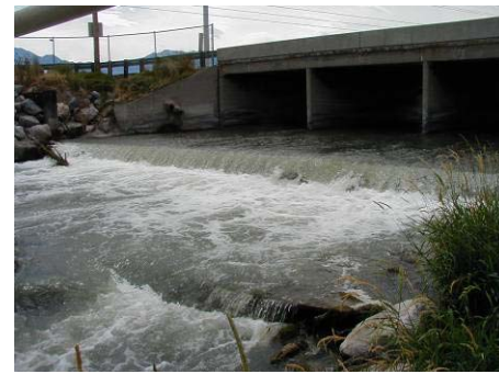
Figure 4.7.2 Pipeline, bridge at 6400 South (WP 9-02)
