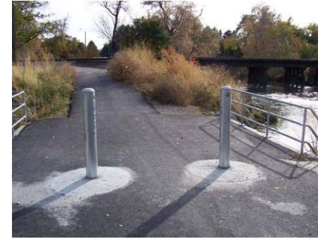
Figure 3.10.44 Trail starting point dead-ends at railroad tracks, south of 900 south
