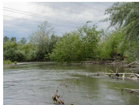
Figure 4.8.7 Fallen tree covers half of channel (WP 9-27)
