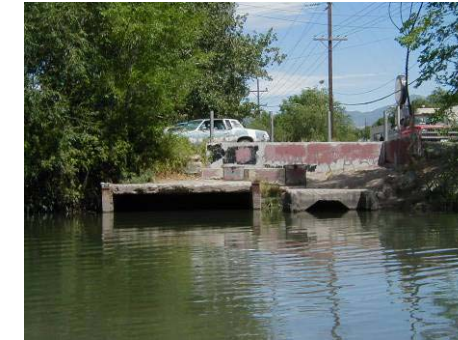
Figure 4.10.5 Storm drain, tributary at 1200 South (WP 11-15)
