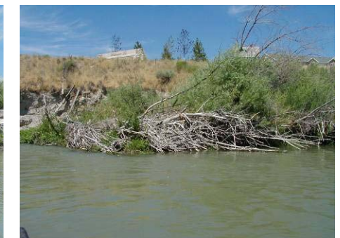
Figure 4.3.14 Tree flood debris north of 12600 South (WP 6-07)
