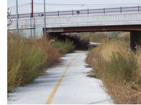
Figure 3.9.54 Pedestrian underpass, 2100 South, looking north
