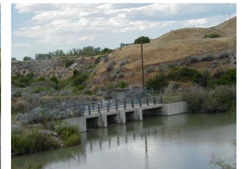
Figure 4.1.23 Take out at Lower Narrows Irrigation Dam (WP 3-25)
