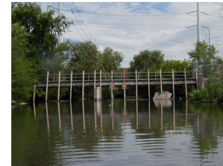
Figure 4.11.9 Rocky Mtn. Power weir with canoe chute at South Temple (WP 12-11)
