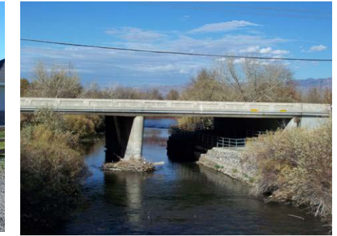
Figure 3.7.33 5400 South vehicular crossing
