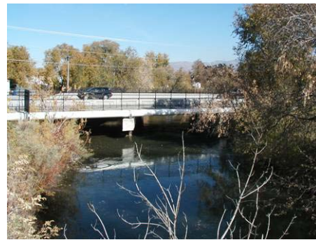
Figure 3.10.19 California Avenue overpass
