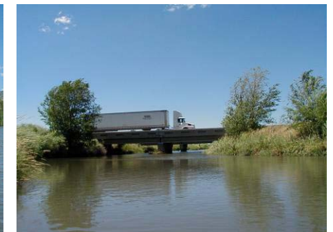
Figure 4.12.18 Vehicular bridge at Interstate 215 North (WP 14-12)
