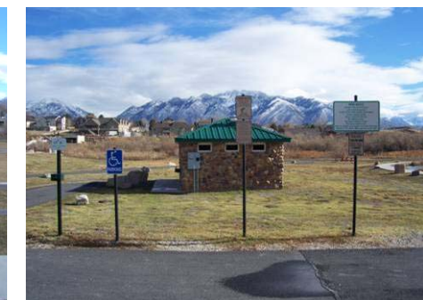
Figure 3.4.16 Riverfront Park signage and restroom facilities
