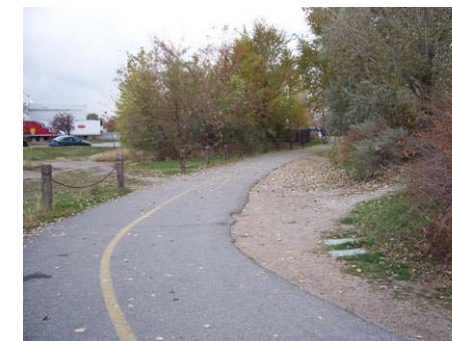
Figure 3.9.13 View to south from east side of Bridge B15
