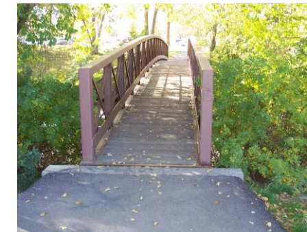
Figure 3.11.10 Bridge B27 4' wide, 70' span, 8' clearance
