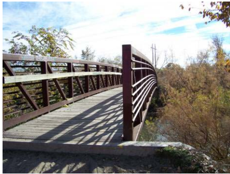
Figure 3.8.20 Bridge B14 8' wide, 105' span, 11' clearance
