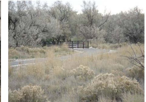
Figure 3.2.11 Footbridge along Spring View Farms Trail
