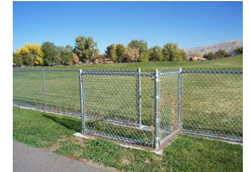
Figure 5.3.6 Trail Access Point
