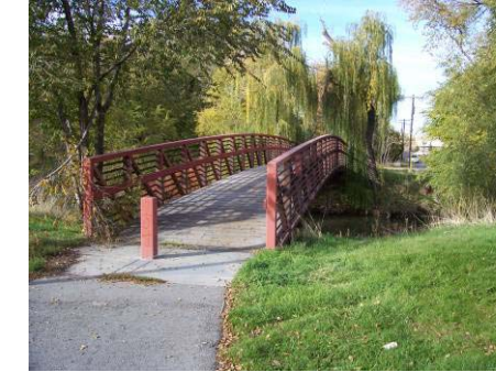
Figure 3.10.50 Bridge B23 10' wide, 100' span, 11' clearance
