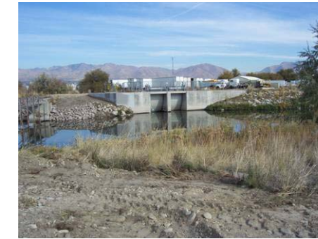
Figure 3.9.56 Diversion Dam near Glendale Golf Course
