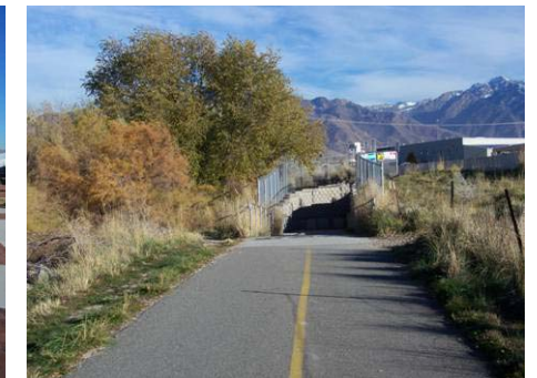
Figure 3.8.13 4700 South pedestrian underpass
