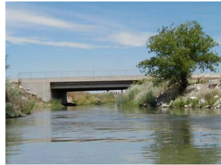
Figure 4.4.7 Bridge at 10600 South, potential launch site (WP 6-17)
