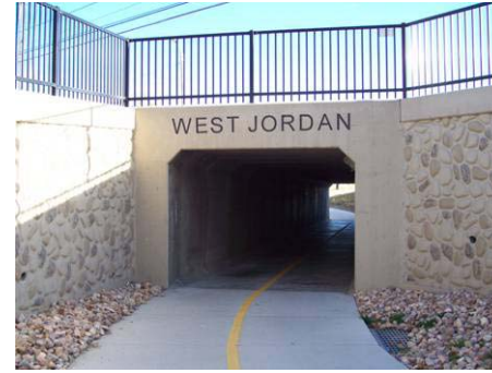
Figure 3.6.50 Winchester Street underpass
