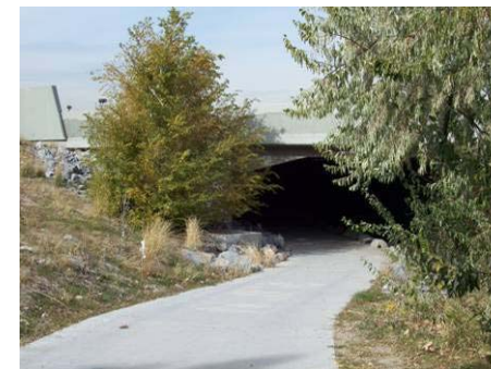
Figure 3.9.53 Pedestrian underpass SR 201
