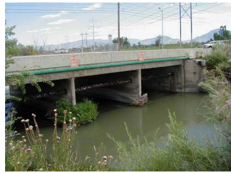
Figure 4.7.1 Vehicular Bridge at 6400 South (WP 9-01)
