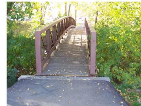
Figure 3.11.10 Bridge B27 4' wide, 70' span, 8' clearance
