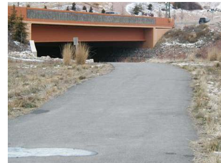
Figure 3.3.22 12300 South underpass, looking south
