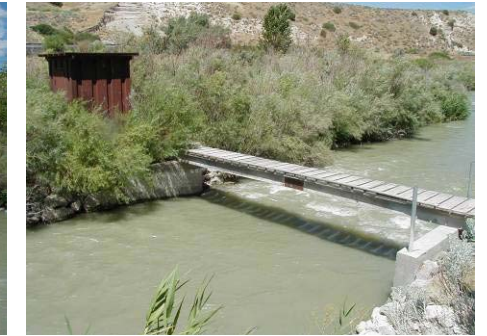
Figure 4.1.5 Foot bridge for Gauging Station Bridge at the Narrows (WP 3-04)
