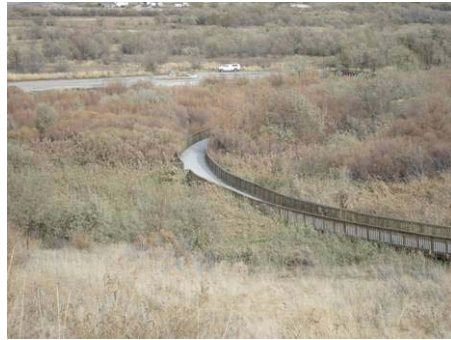
Figure 3.3.17 Boardwalk winding through the wetlands
