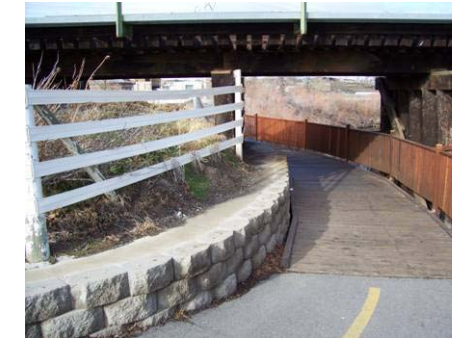
Figure 3.6.33 Railroad Bridge underpass
