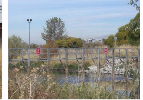
Figure 3.9.55 Maintenance access footbridge north of 2100 south, no public access
