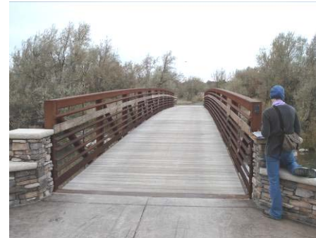
Figure 3.2.2 Bridge B1 10' wide, 100' span, 6' clearance
