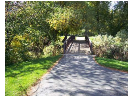
Figure 3.11.25 Bridge B28 8' wide, 70' span, 8' clearance
