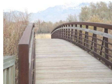
Figure 3.3.2 Bridge B3 8' wide, 130' span, 10' clearance
