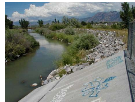
Figure 4.5.7 Launch north side of 9600 South dam (WP 7-09)
