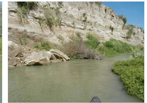
Figure 4.3.12 Flood debris, boulders from slumps (WP 6-05)
