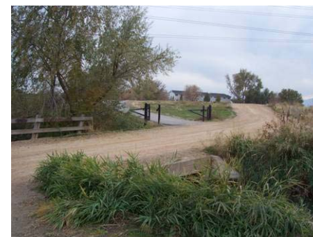
Figure 3.9.32 Trail Crossing west of Power Substation
