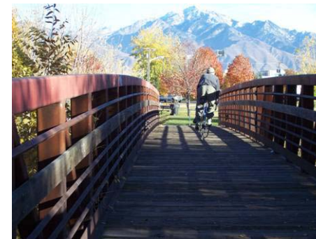
Figure 3.8.6 Bridge B13 8' wide, 92' span, 14' clearance
