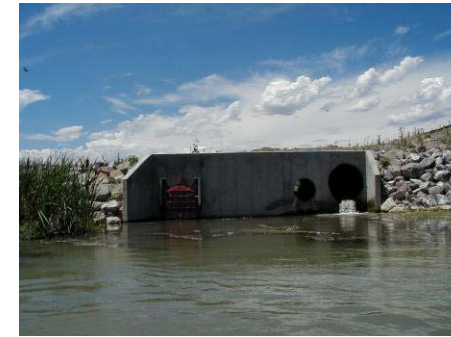
Figure 4.4.8 Vehicular bridge at 10600 South (WP 6-18)
