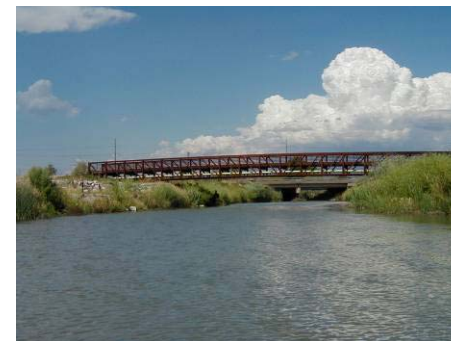
Figure 4.5.9 River Oaks Golf Course footbridge (WP 7-11)
