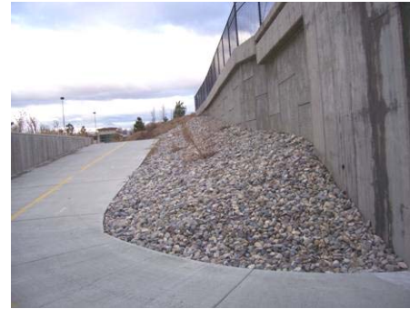
Figure 3.4.27 View to west from 10600 South underpass
