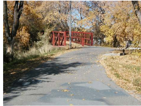
Figure 3.10.17 Bench near Bridge B19
