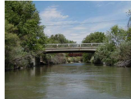
Figure 4.8.2 Vehicular and foot bridges at 4800 South (WP 9-20)
