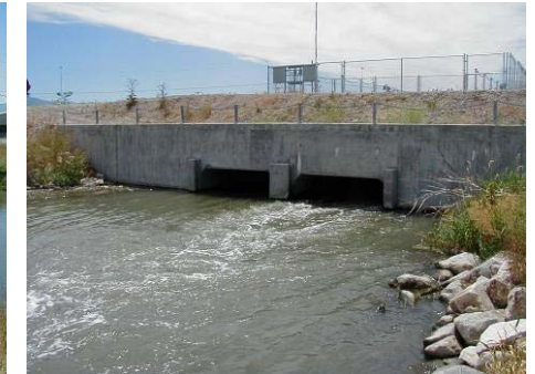
Figure 4.9.8 Diversion dam at 2100 South downstream (WP 10-13)
