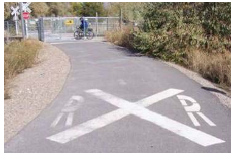
Figure 3.9.64 Gated railroad crossing for bikes and pedestrians
