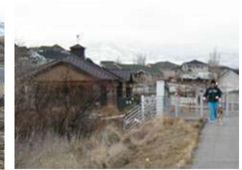
Figure 3.3.33 Bridge B4, looking west at Dr. O. Roi Hardy Park
