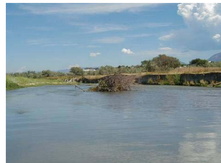
Figure 4.4.2 Flood debris in middle of channel (WP 6-12)
