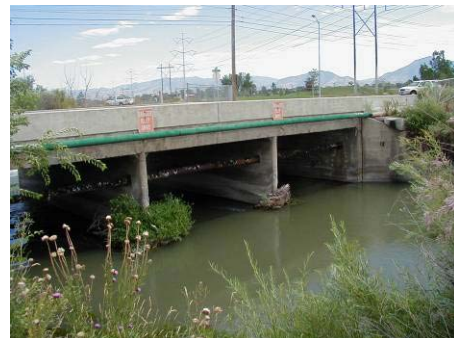
Figure 4.7.1 Vehicular Bridge at 6400 South (WP 9-01)
