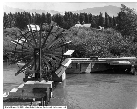
Figure 1.2 Water wheel on Jordan River, 1914
