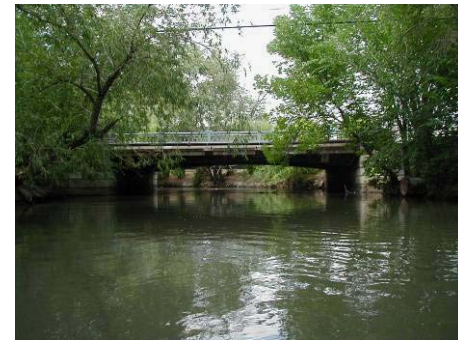
Figure 3.10.18 Vehicular bridge at 300 South (WP 11-31)
