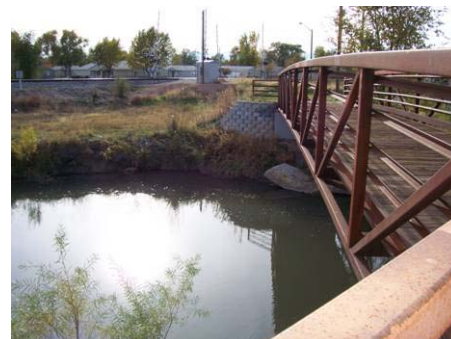
Figure 3.10.48 Bridge B22 10' wide, 70' span, 10' clearance
