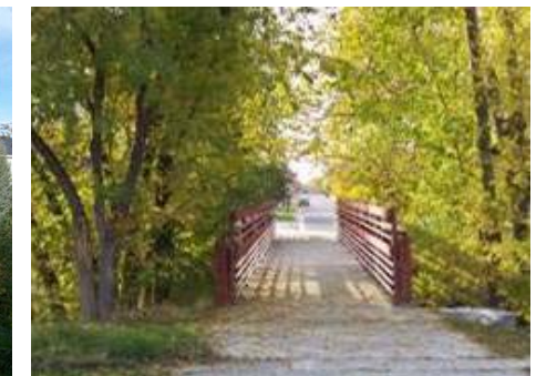
Figure 3.10.53 Bridge B24 7' wide, 77' span, 6' clearance
