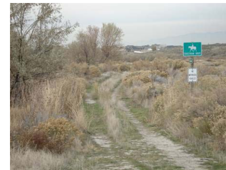
Figure 3.3.8 Equestrian trail beginning at culvert, looking northeast
