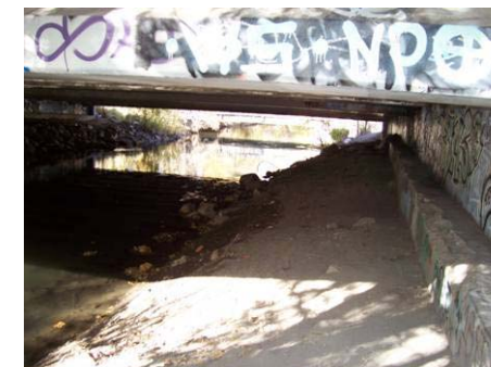
Figure 3.10.69 View under Interstate 80 overpass
