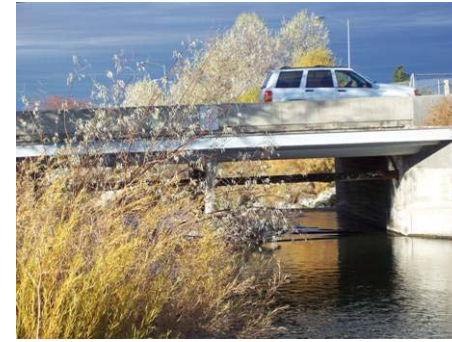
Figure 3.6.51 Winchester Street river crossing, looking north
