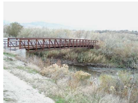
Figure 3.3.1 Bridge B2 6' wide, 90' span, 20' clearance
