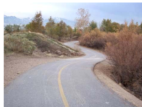
Figure 3.9.24 Trail looking north, near Bridge B15
