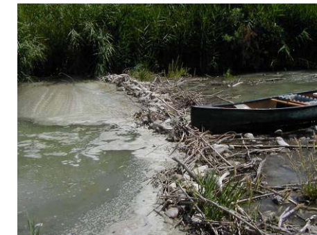
Figure 4.2.11 Rock weir (WP 4-21)
