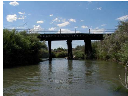
Figure 4.6.6 Railroad crossing bridge (WP 8-07)
