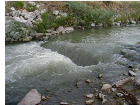
Figure 4.6.3 Qwest fiber-optic pipeline before bridge (WP 8-04)
