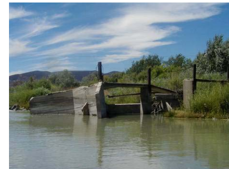
Figure 4.2.3 Cultural Site, Historic Dam (WP 4-13)
