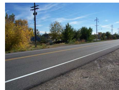
Figure 3.12.11 Redwood Road crossing, looking southeast
