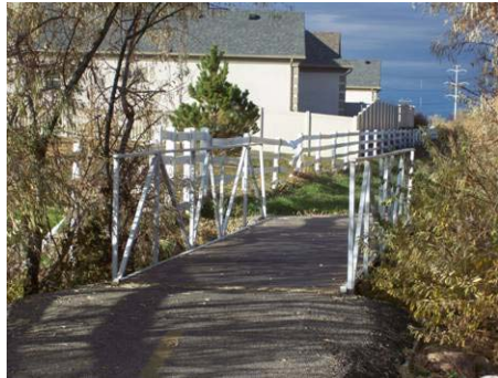
Figure 3.6.41 Footbridge north of 7000 South
