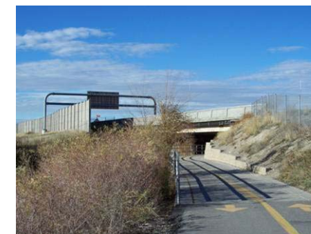
Figure 3.7.16 Interstate 215 pedestrian underpass, looking north
