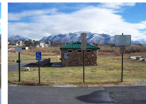
Figure 3.4.16 Riverfront Park signage and restroom facilities
