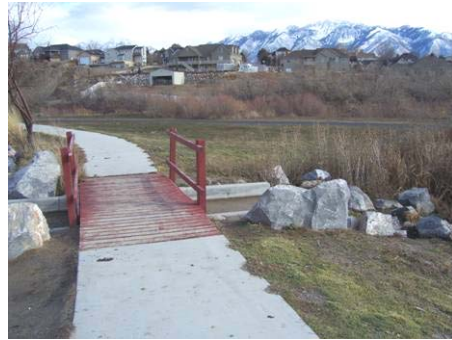
Figure 3.4.19 Footbridge in Riverfront Park
