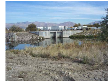
Figure 3.9.56 Diversion Dam near Glendale Golf Course
