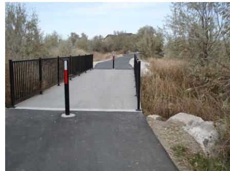
Figure 3.2.6 Footbridge along Jordan River Trail
