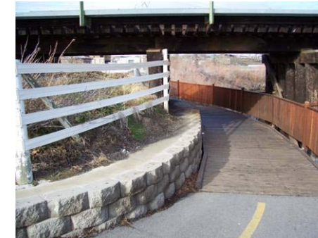
Figure 3.6.33 Railroad Bridge underpass
