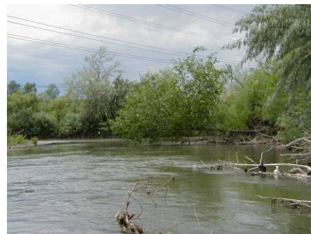
Figure 4.8.7 Fallen tree covers half of channel (WP 9-27)
