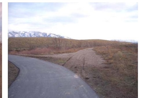
Figure 3.6.16 View to south, west of Bridge B8, looking toward unpaved portion of trail
