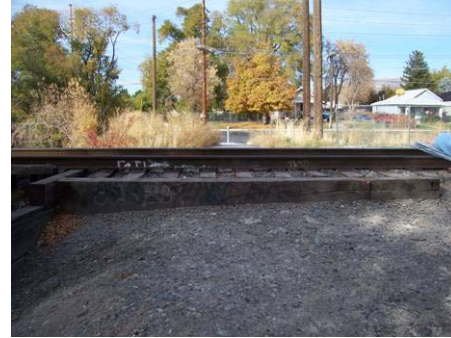
Figure 3.10.43 Non-accessible railroad crossing south of 900 South
