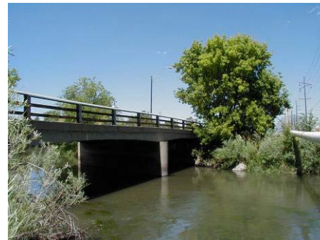
Figure 4.12.7 Vehicular bridge at Redwood Road (WP 13-10)
