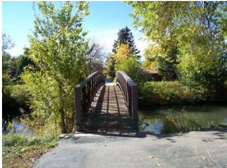
Figure 3.11.37 Bridge B30 4' wide, 70' span, 6' clearance
