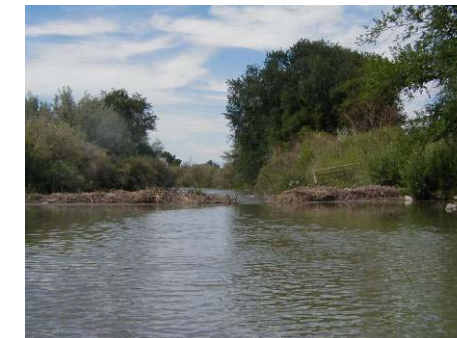
Figure 4.2.13 Earthen weir (WP 4-27)
