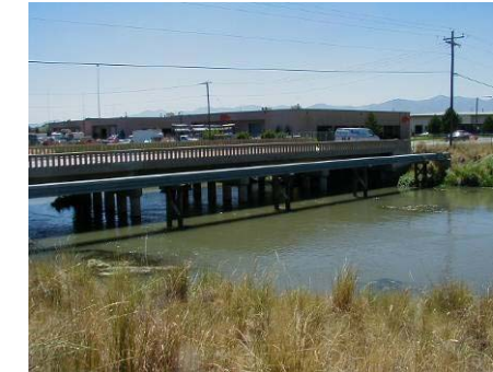
Figure 4.9.7 Pipeline across river near 2100 South (WP 10-12)
