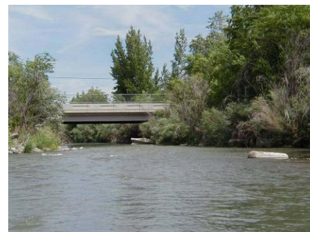
Figure 4.7.9 Vehicular bridge at Bouillon Street (WP 9-10)
