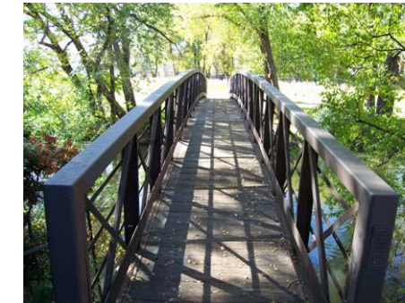
Figure 3.11.30 Bridge B29 4' wide, 69' span, 6' clearance
