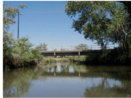
Figure 4.12.1 Bridge at Rose Park Golf Course (WP 13-03)
