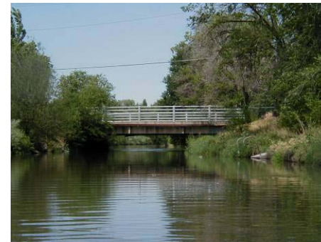
Figure 4.11.24 Vehicular bridge at 1000 North (WP 12-38)
