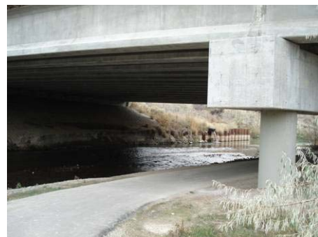
Figure 3.2.22 Bangerter Highway Underpass
