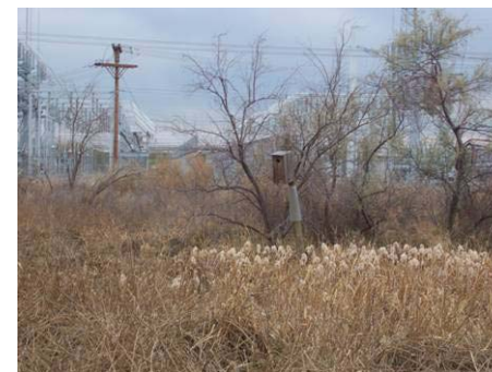
Figure 3.9.30 Nesting box near Power Substation
