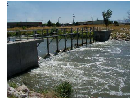
Figure 4.9.11 Weir at surplus canal at 2100 South (WP 10-16)
