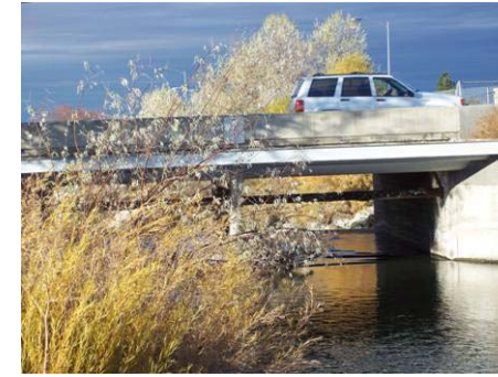
Figure 3.6.51 Winchester Street river crossing, looking north
