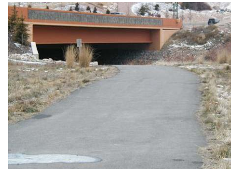
Figure 3.3.22 12300 South underpass, looking south
