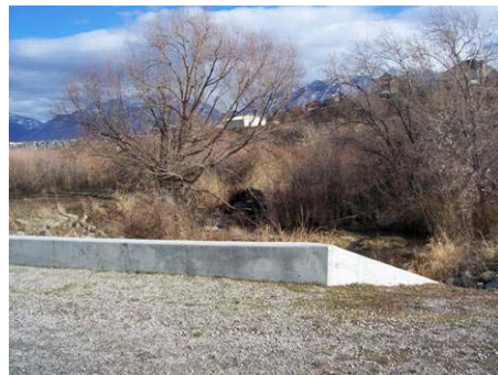
Figure 3.4.21 Footbridge crossing small stream
