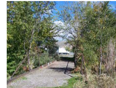
Figure 3.12.16 Bridge B32 8.5' wide, 88' span, 6' clearance
