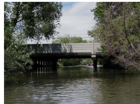
Figure 4.10.2 Vehicular bridge at 1700 South (WP 11-09)
