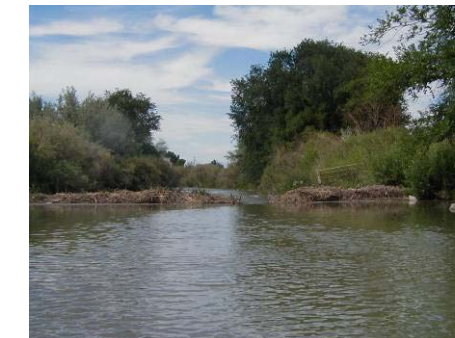
Figure 4.2.13 Earthen weir (WP 4-27)
