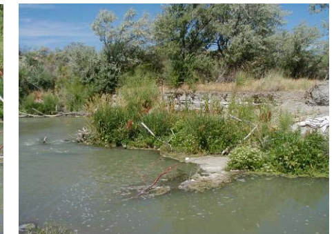
Figure 4.3.10 Slumping bank (WP 6-03)
