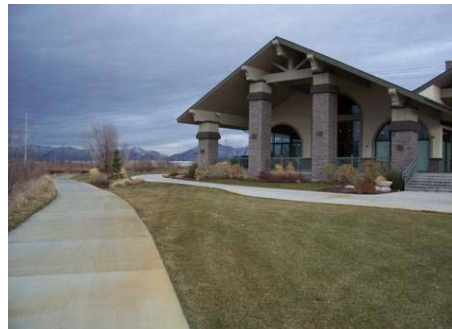
Figure 3.5.21 View from trail near River Oaks Golf Course Club House, looking north
