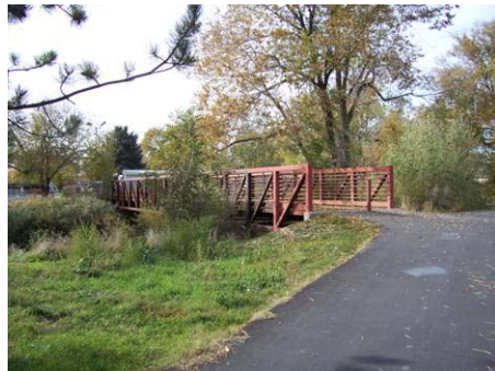
Figure 3.10.37 Bridge B21 10' wide, 100' span, 6' clearance
