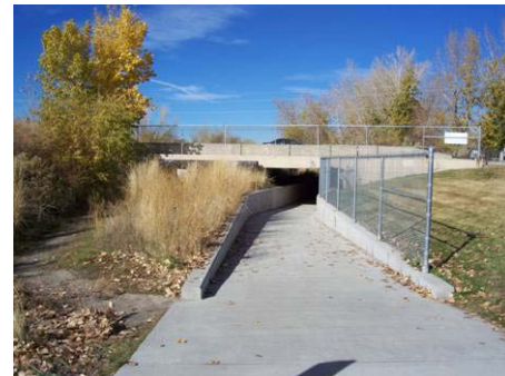
Figure 3.9.2 3500 South pedestrian underpass, looking north
