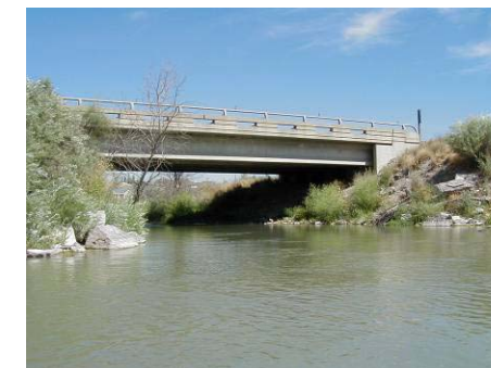
Figure 4.3.13 Vehicular bridge at 12600 South (WP 6-06)
