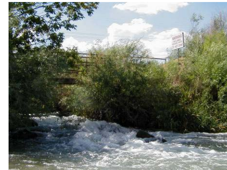
Figure 4.6.7 Sewage plant discharge at 7400 South (WP 8-08)
