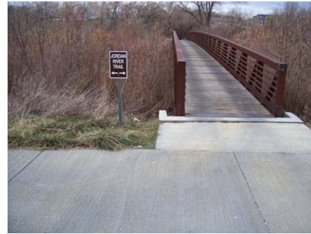
Figure 3.5.25 Bridge B6 6' wide, 130' span, 8' clearance
