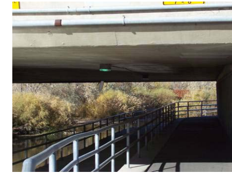
Figure 3.7.34 5400 South pedestrian and equestrian underpass
