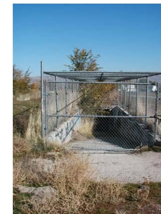
Figure 3.10.12 Utility Structure near informal Labyrinth path
