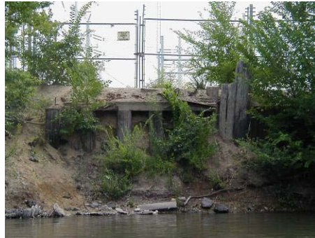
Figure 4.11.11 Old trestle piers (WP 12-13)
