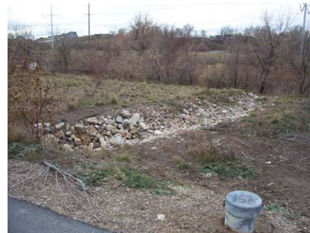
Figure 3.6.7 Stone-lined drainage swale along trail
