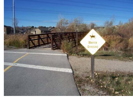
Figure 3.7.50 Bridge B12 8' wide, 122' span, 8' clearance
