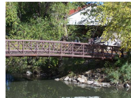
Figure 3.11.8 Bridge B26 8' wide, 77' span, 9' clearance
