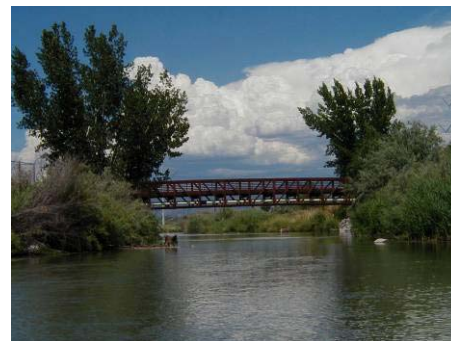
Figure 4.5.8 River Oaks Golf Course footbridge (WP 7-10)
