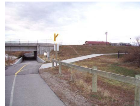
Figure 3.4.30 Trail connection to 10600 South near Mulligan's Golf
