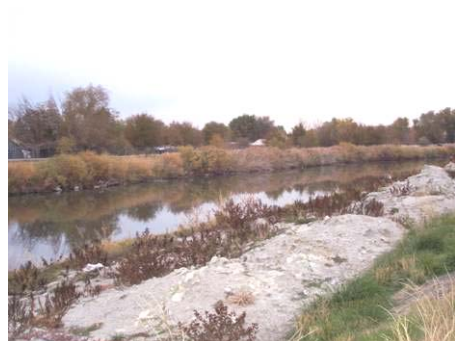
Figure 3.9.21 View to northwest, near Redwood Nature Area
